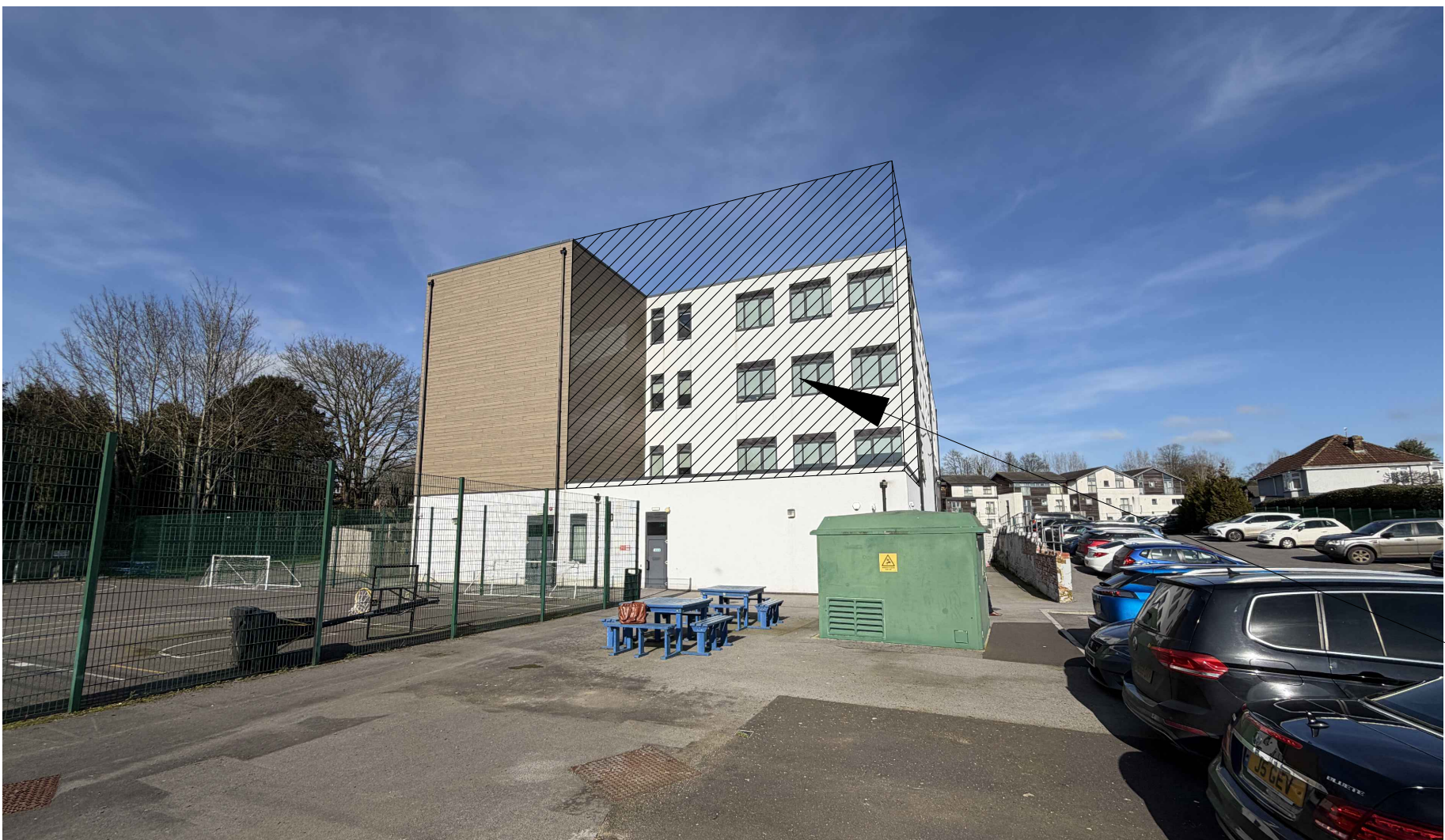
EXISTING BUILDING SOUTH ELEVATION
