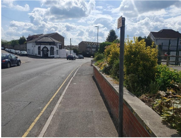
Photo 2: Footway on Western Side of Tollgate Road
