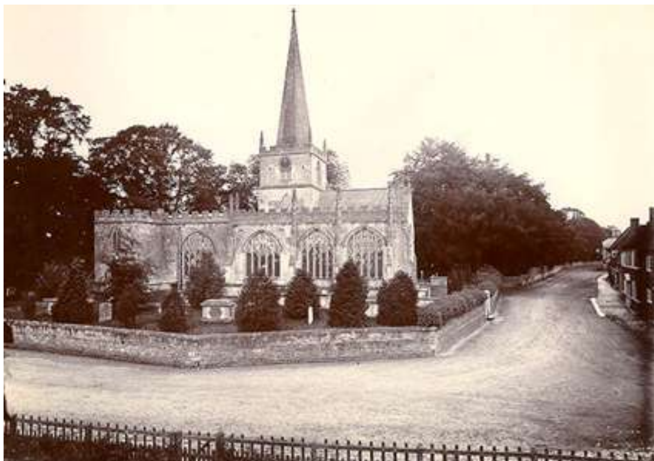
Figure 6 : Photograph of the Grade I Listed St Nicholas Church Nearby in Bromham.
