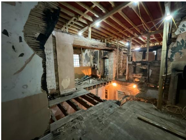
Figure 4: Underside of the temporary roof at second floor
