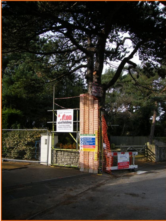
Pictures 4 & 5: Wooden boards carefully secured around the trunks can provide good protection where access is limited.
