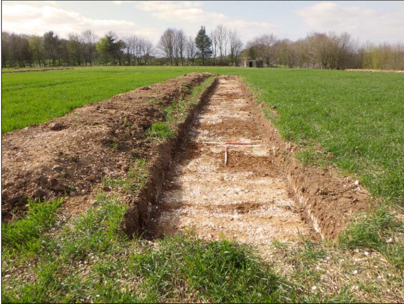
Plate 1: Trench 2, view to northwest (2 x 1m scale)
