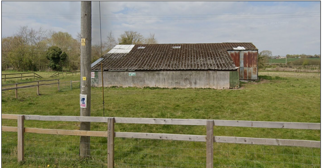
Figure 5 – The Existing Building Viewed from the Road
