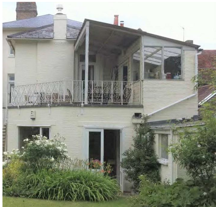
Rear showing 1964 extension
