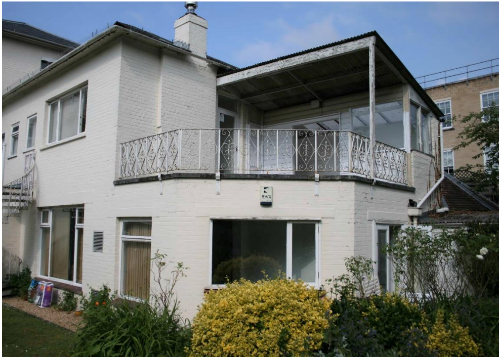
1854 Building with 1964 extension
