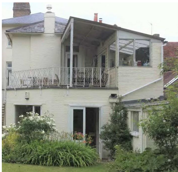
Photo 2 Existing Rear Elevation
