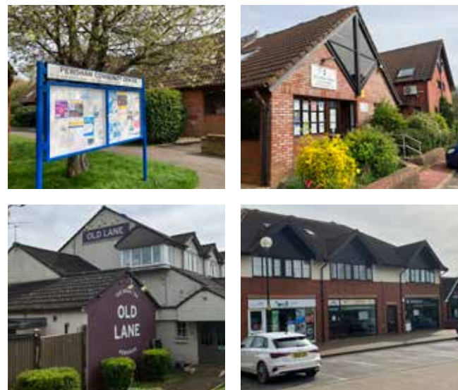
Figure 4.12 Cluster of facilities at Pewsham
