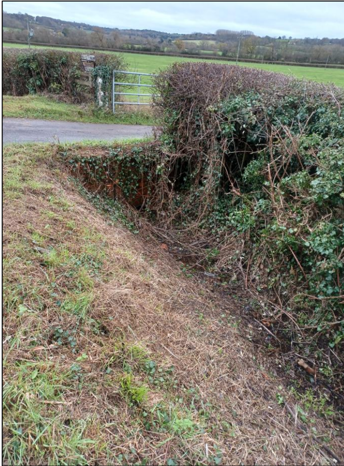
Figure 5.2: Upstream side of ditch culvert underneath existing access
