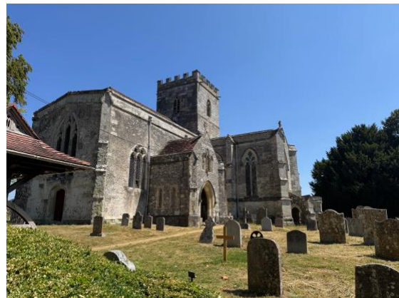
St John the Baptist Church, Bishopstone. The footpath can be seen in this picture and the one below.
