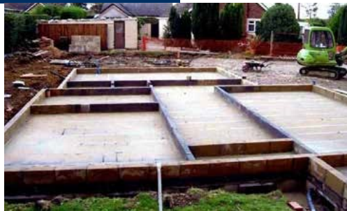
Upstands must be dense concrete blocks or concrete. These are built to the same height as the finished floor for external and internal walls.
