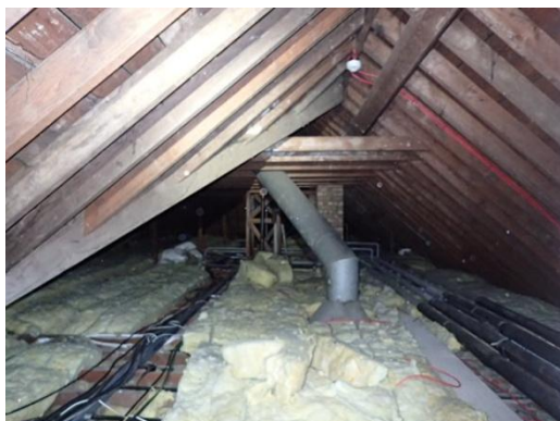
Figure 2.6. The open roof void
