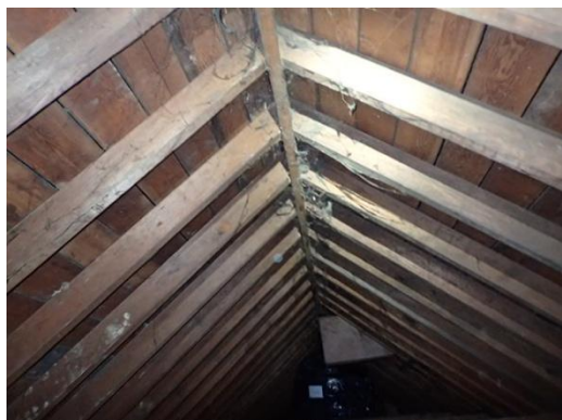
Figure 2.7. The roof lining
