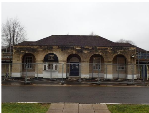
Figure 2.2. The north elevation of the building
