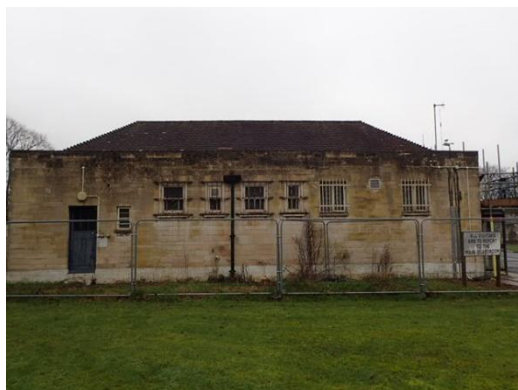
Figure 2.5. The west elevation of the building
