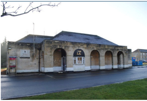
Façade (Northeast Elevation), 2020
