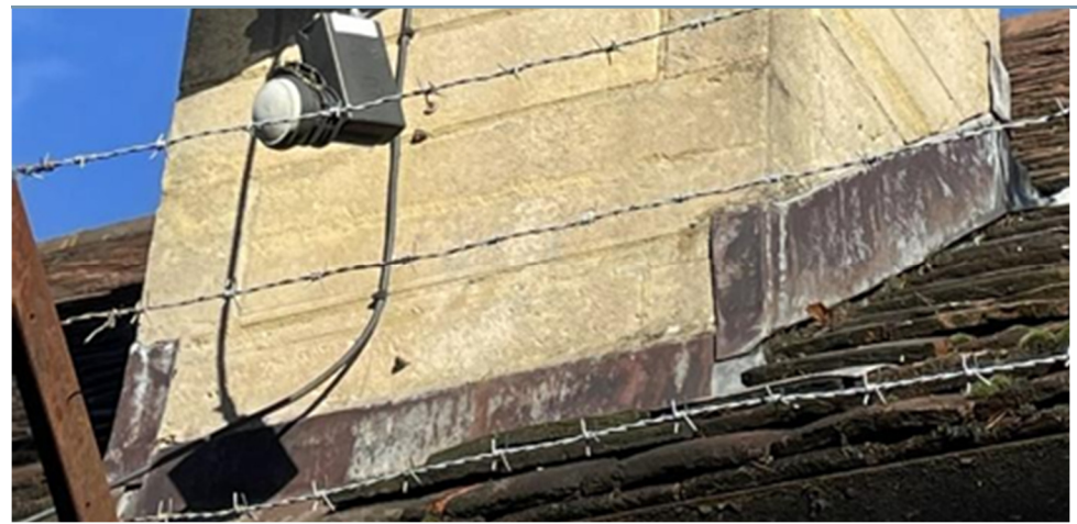
Chimney Stack Front and Side Flashing, 2026
