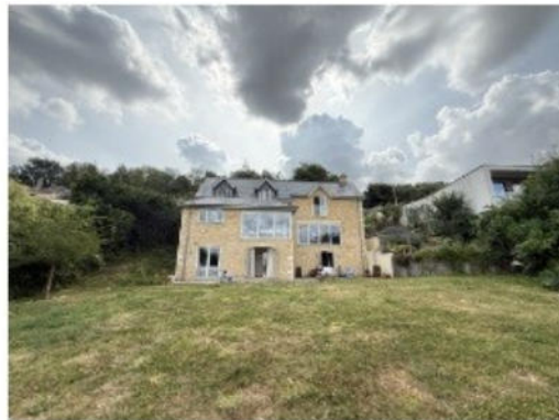
View on B: Rear elevation of property
