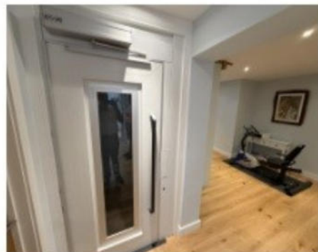
View B: Lift shaft and basement hallway area
