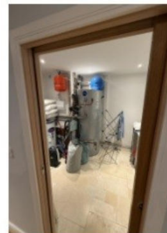
View G: Existing Plant room/utility from lower hall
