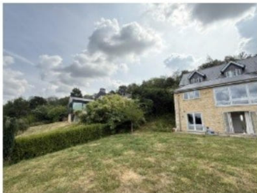
View on C: Left hand side of property with new rebuilt property to left plot as viewed from right
