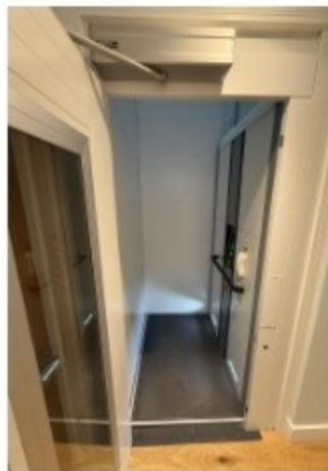
View E: Lift door opened at basement level
