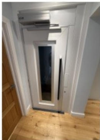
View A: Lift shaft in basement hall
