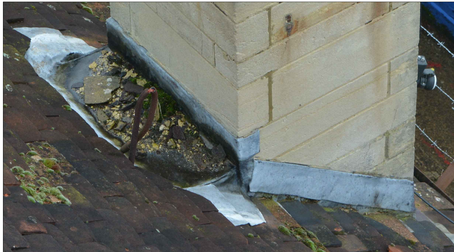
Existing Chimney rear flashing elevation (Scale NTS)
