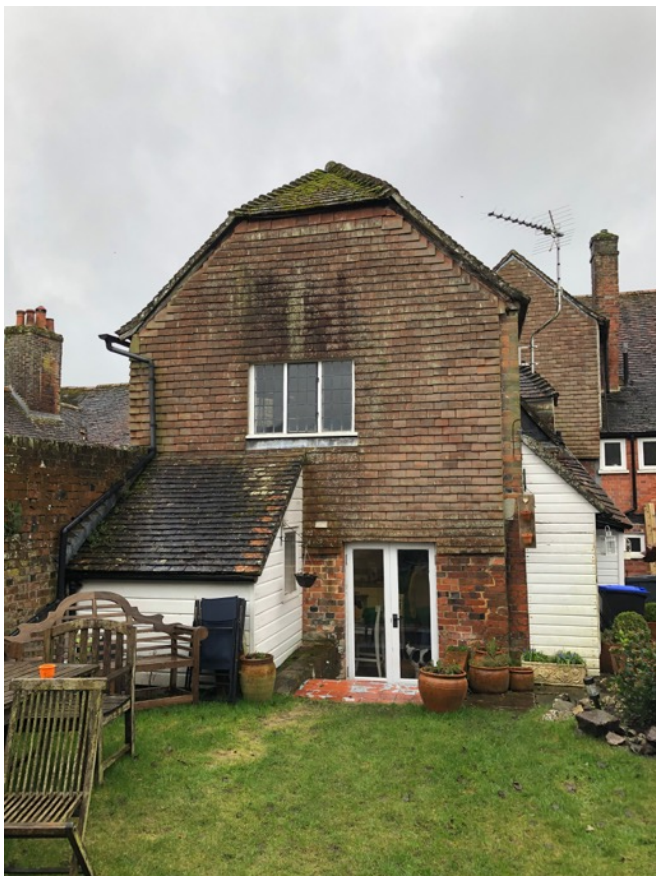
Photo 4 View of rear elevation from the garden
