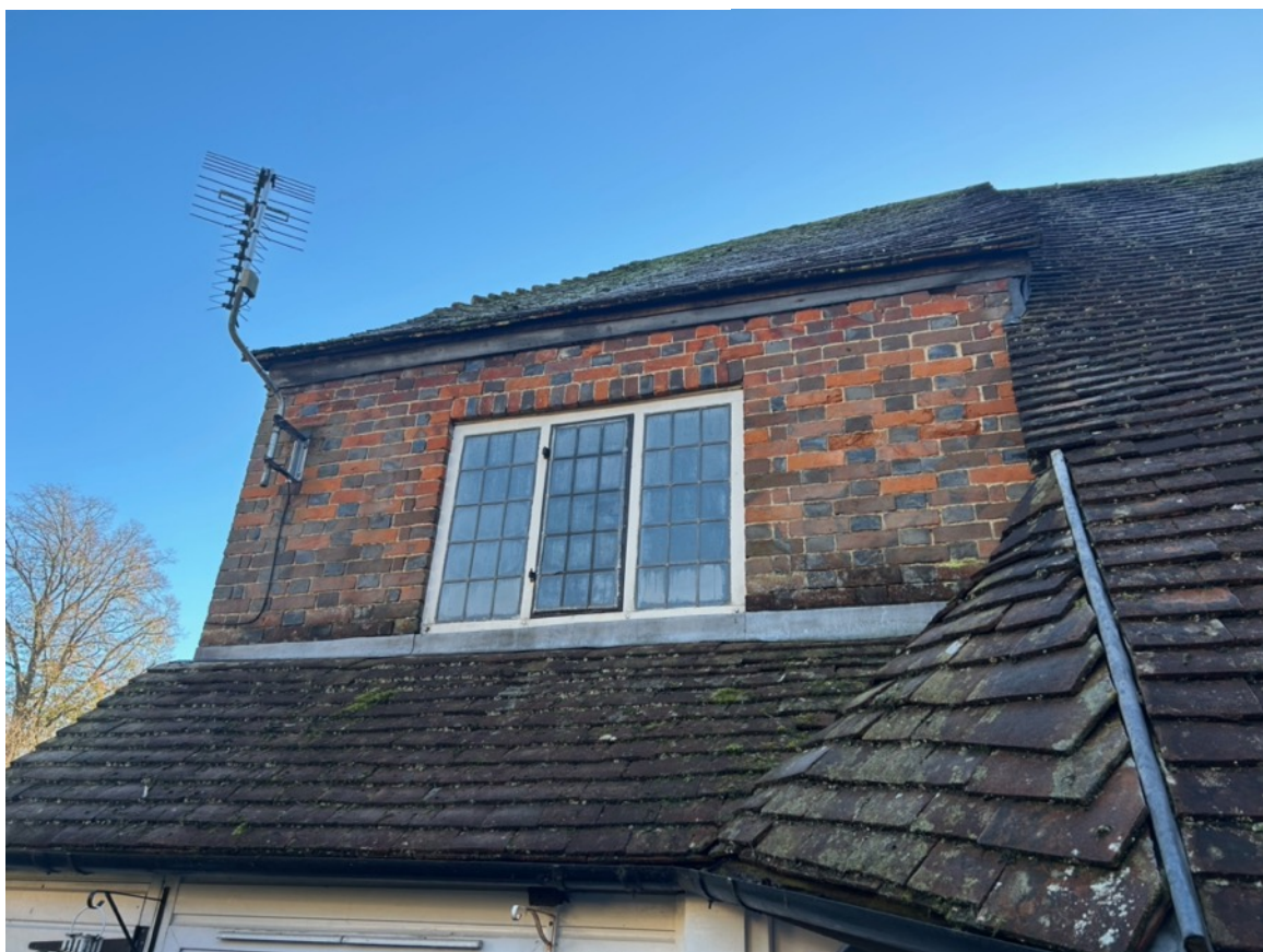
Photo 2 View of existing brickwork to the rear
