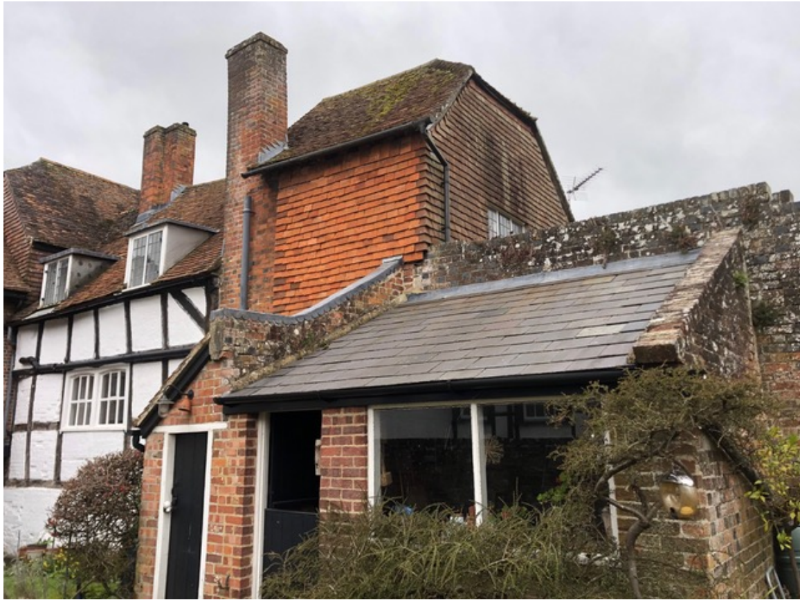
Photo 5 - View of the side elevation chimneys
