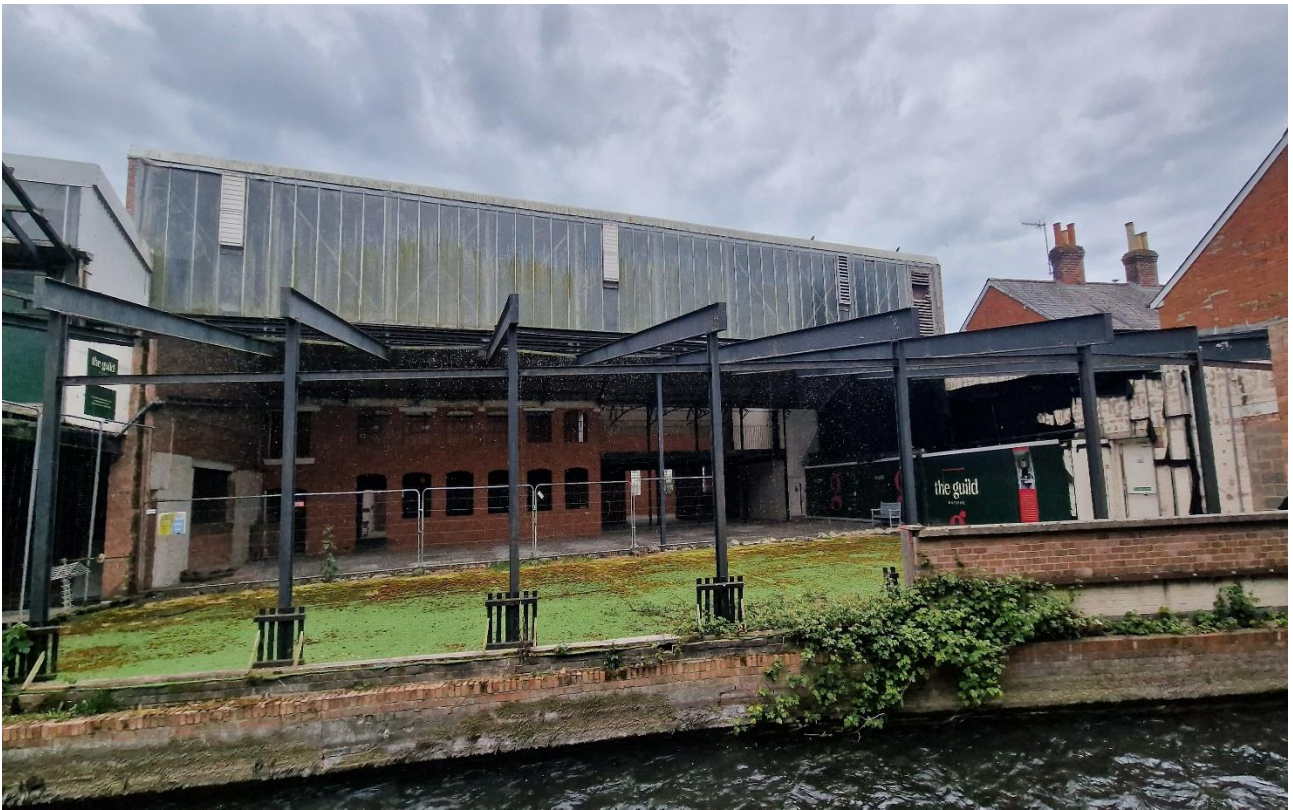
Picture 1: The northern elevation of Unit 5
