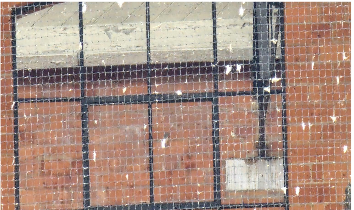
Picture 6: Internal view of Unit 5
