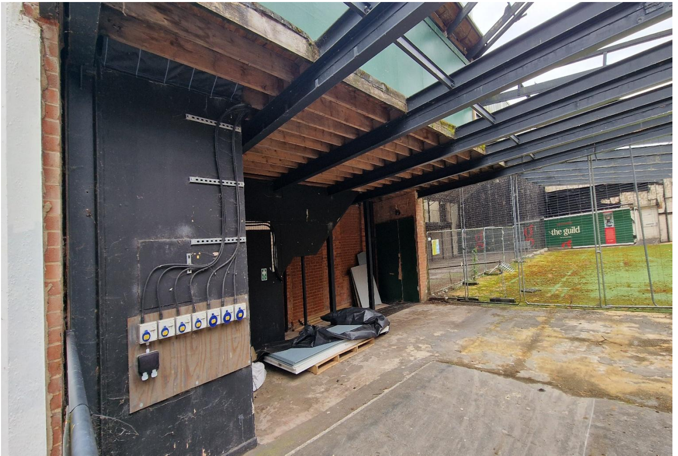
Picture 5: Internal view of Unit 5
