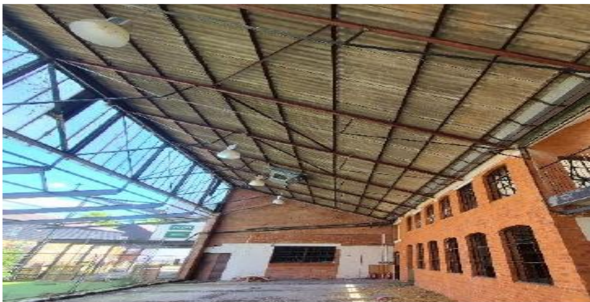
Picture 7: Internal view of Unit 5
