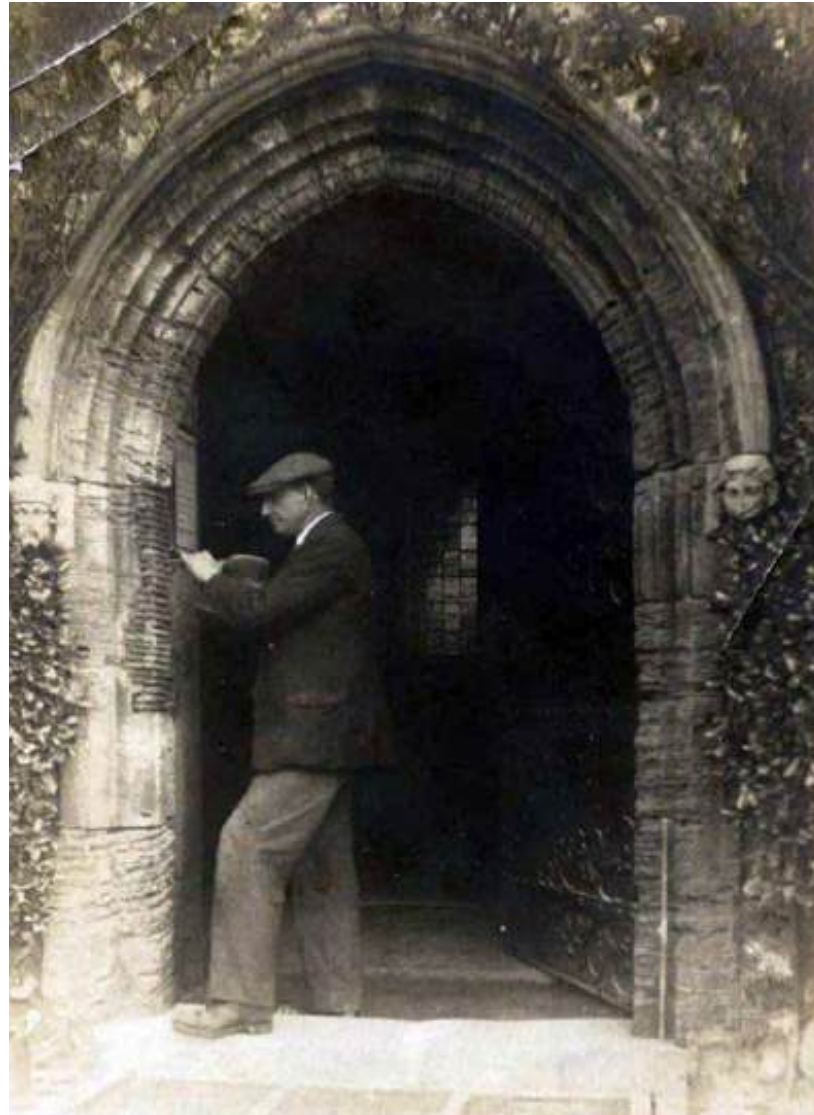
Tile repair to the door of Rottingdean Church, Sussex, 1920s Picture: SPAB
