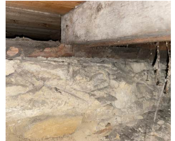
Soft wood floor joists supporting suspended floor in R006 / R007 supported on sleeper walls
