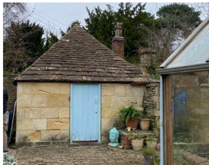
Existing stone outbuilding as existing today
