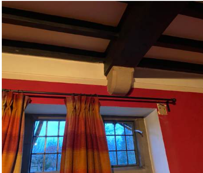
Image locating inspection hole adjacent to window for removal / sliding doors installation
