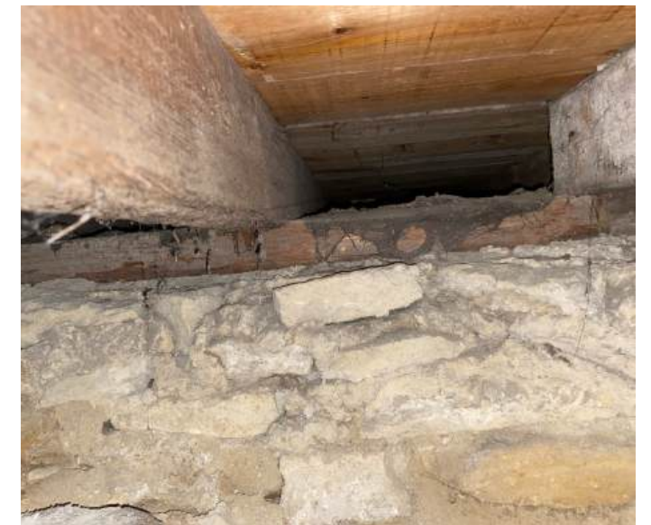
Sleeper wall for supporting floor joist spans R006 / R007
