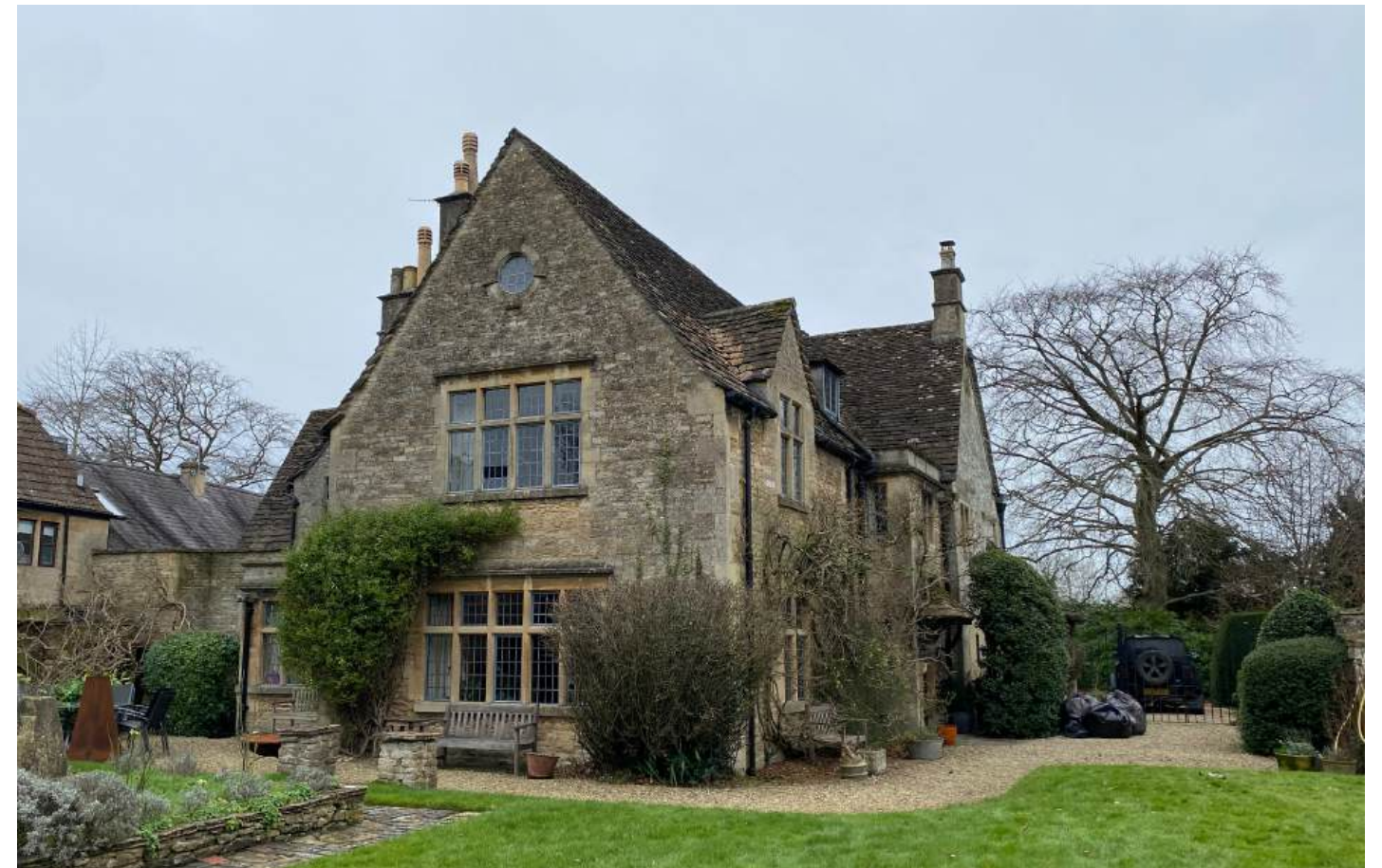
Site photo - South elevation
