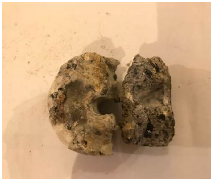
Core sample from R001 - Concrete slab in R001 to be removed and replaced with limecrete construction
