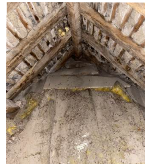
South West Wing - emergency repairs using expanding foam.
