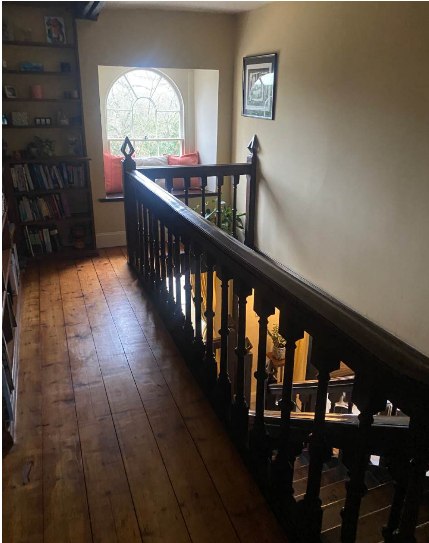
View 3 - Existing arts and craft staircase - For proposed renovation / repositioning
