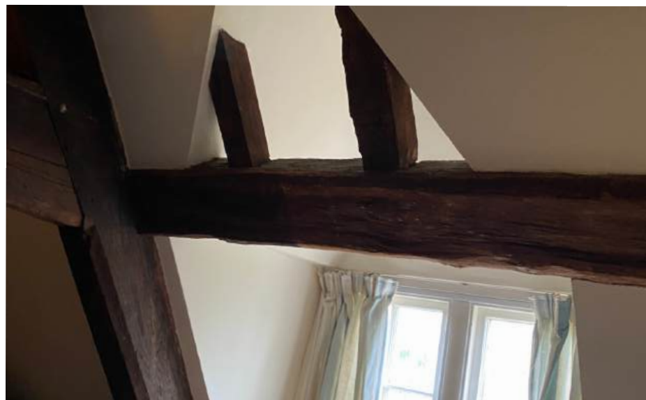
The North (Front) wing roof has a very old roof structure, but modern plasterboarded interior
