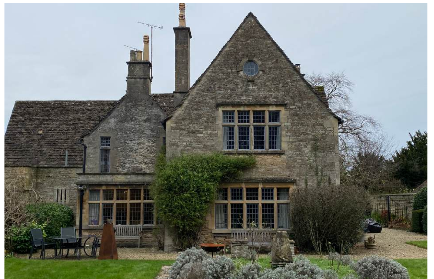
Site photo - South elevation
