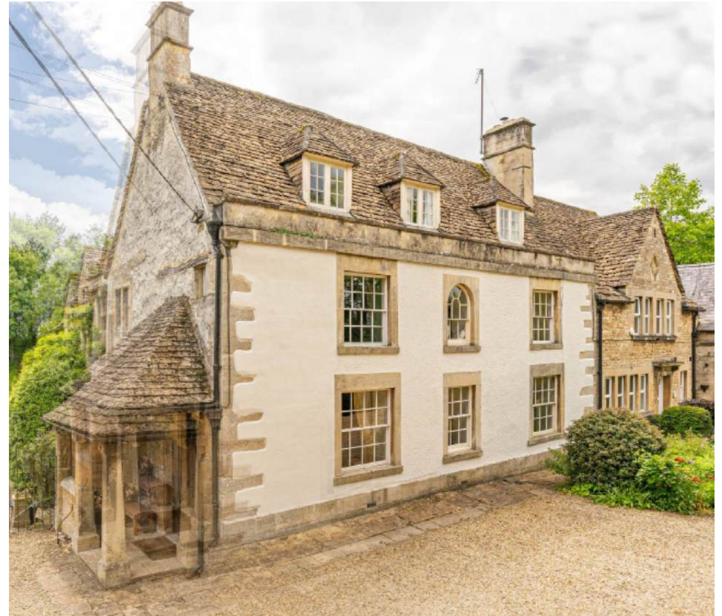
Site photo - North elevation showing 'Gentrified facade' with sash windows - See also three dormers above.
