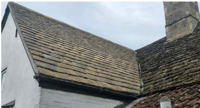
No. 40 Shurnhold - Adjoining Roof/Tiles
