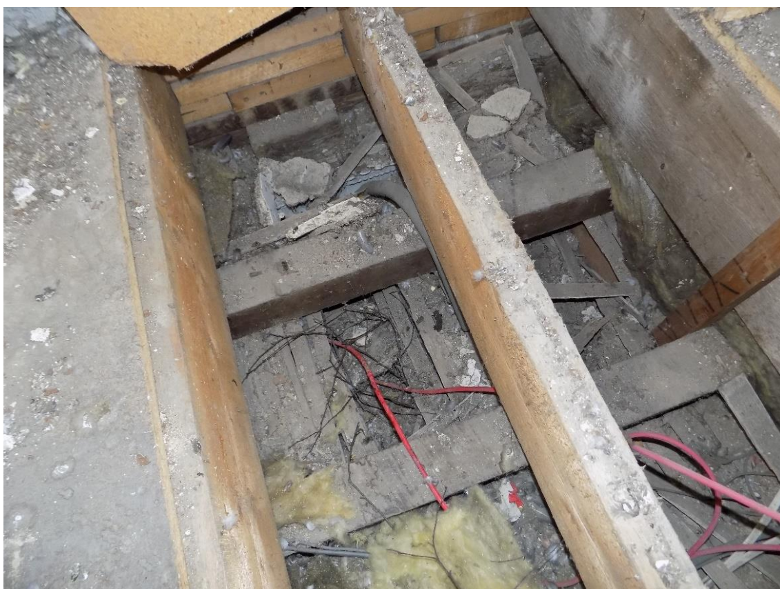
Fig.25: Detail showing oak floor joists beneath the first-floor modern false floor.
