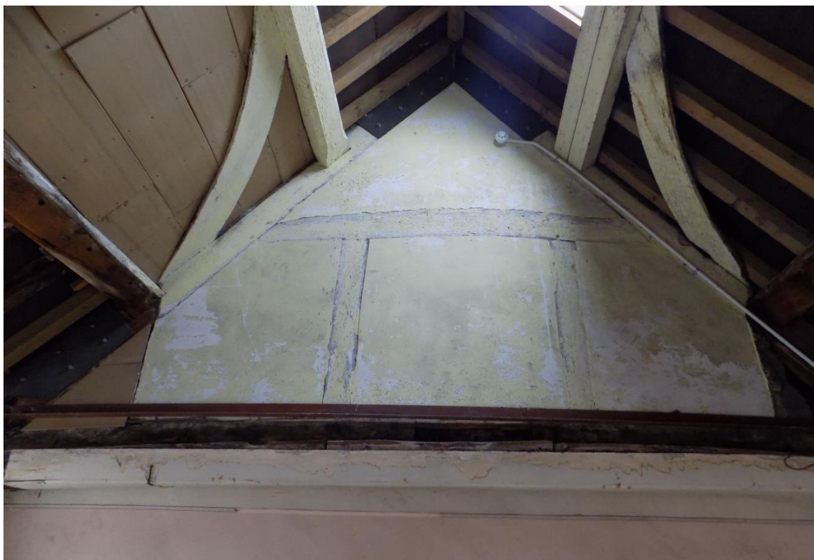
Fig.36: Attic detail showing queen-post collar truss at east end.
