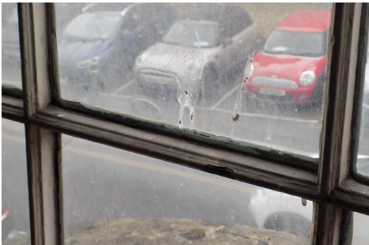
Fig.34: Front-facing window detail showing narrow (c.15mm) ovolo and cavetto glazing bars and bubble in hand-made glass.
