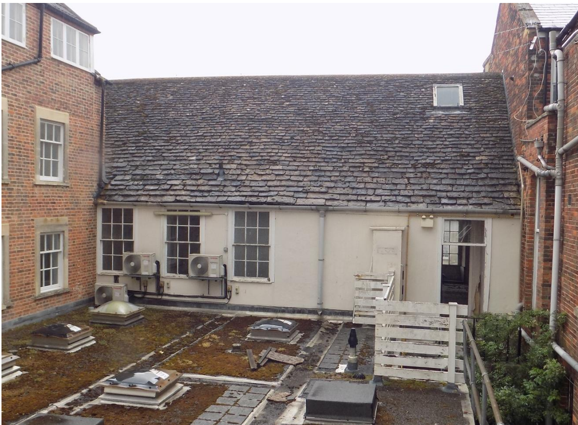
Fig.13: View of the rear of the frontage of No.3 Fore Street, showing inserted door and rooflight.
