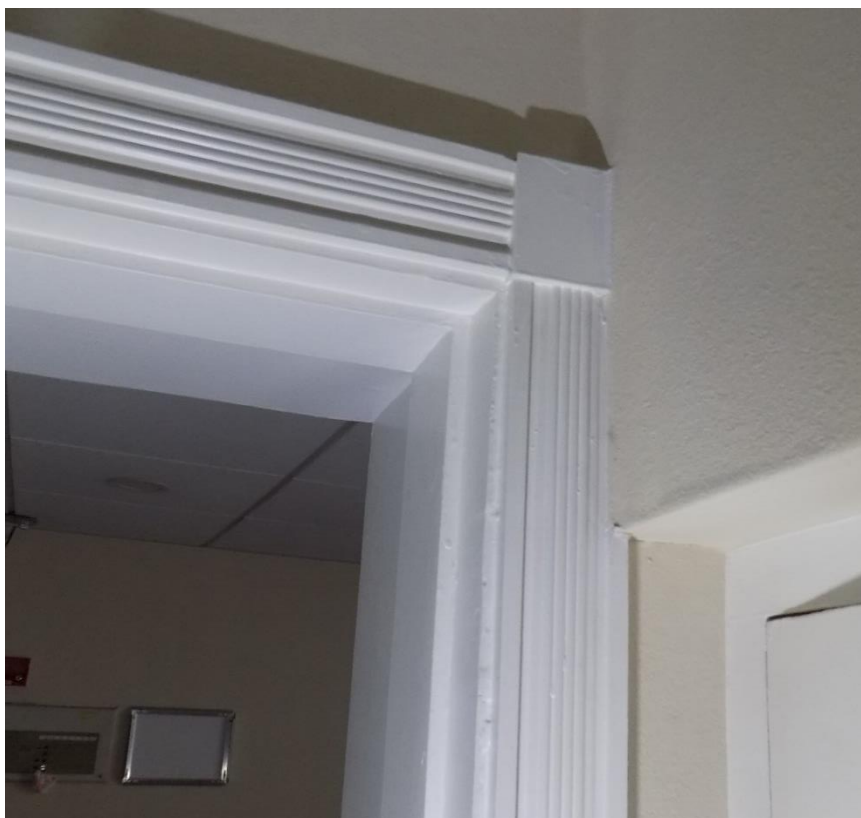
Fig.20: Detail of ground-floor door opening with reeded architraves with corner blocks.
