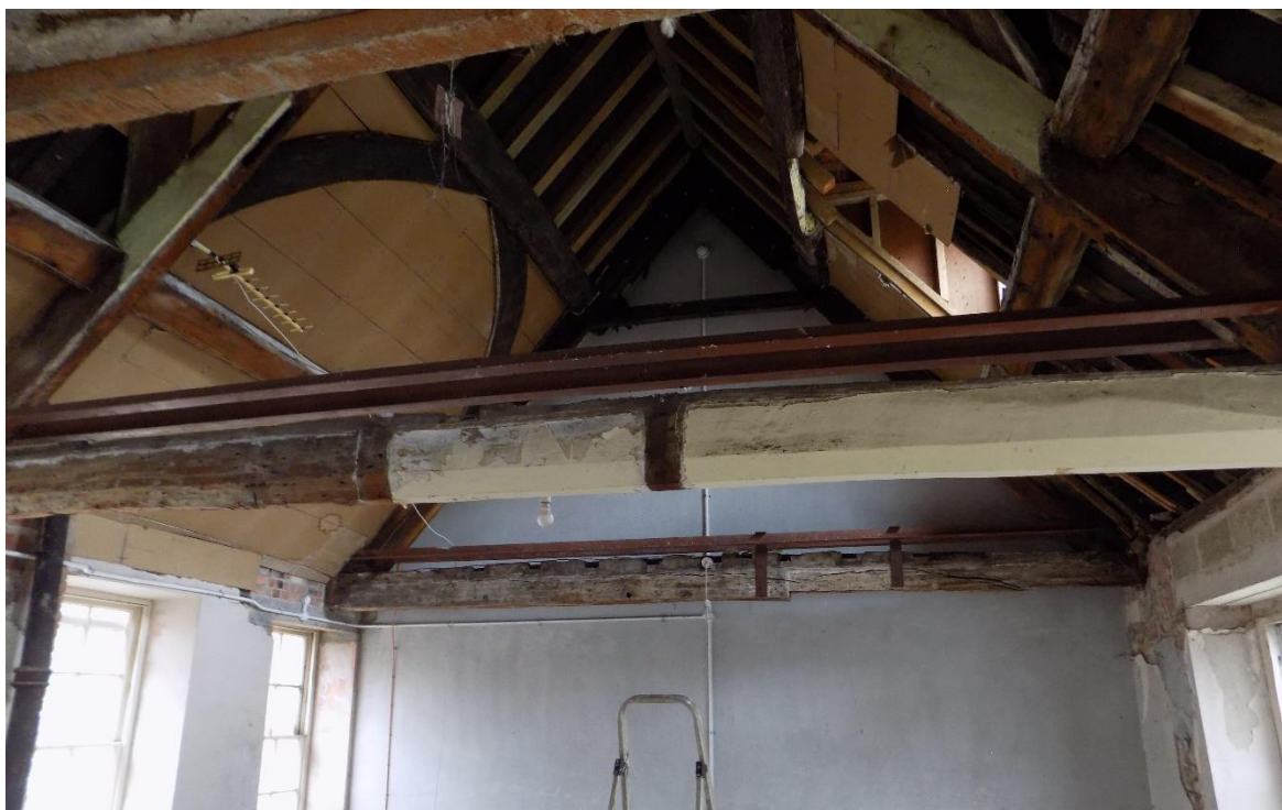
Fig.40: Attic view looking west, showing second tie from east notched for joists at northern end only.
