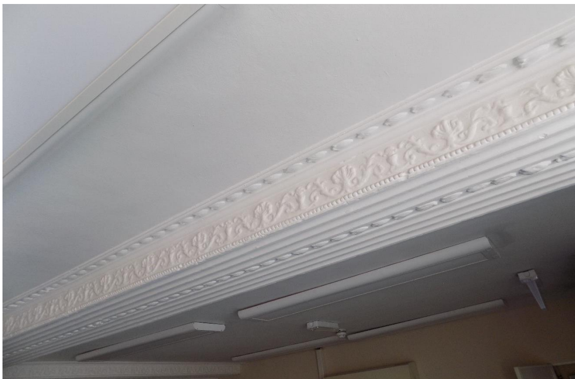
Fig.18: Detail of early eighteenth-century mouldings to beams in ground-floor frontage range.
