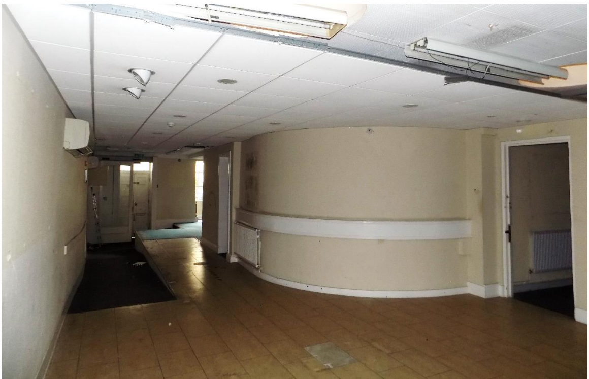
Fig.17: Interior view of the modern rear extension, looking north, with western side of central projecting bay (former external rear wall).
