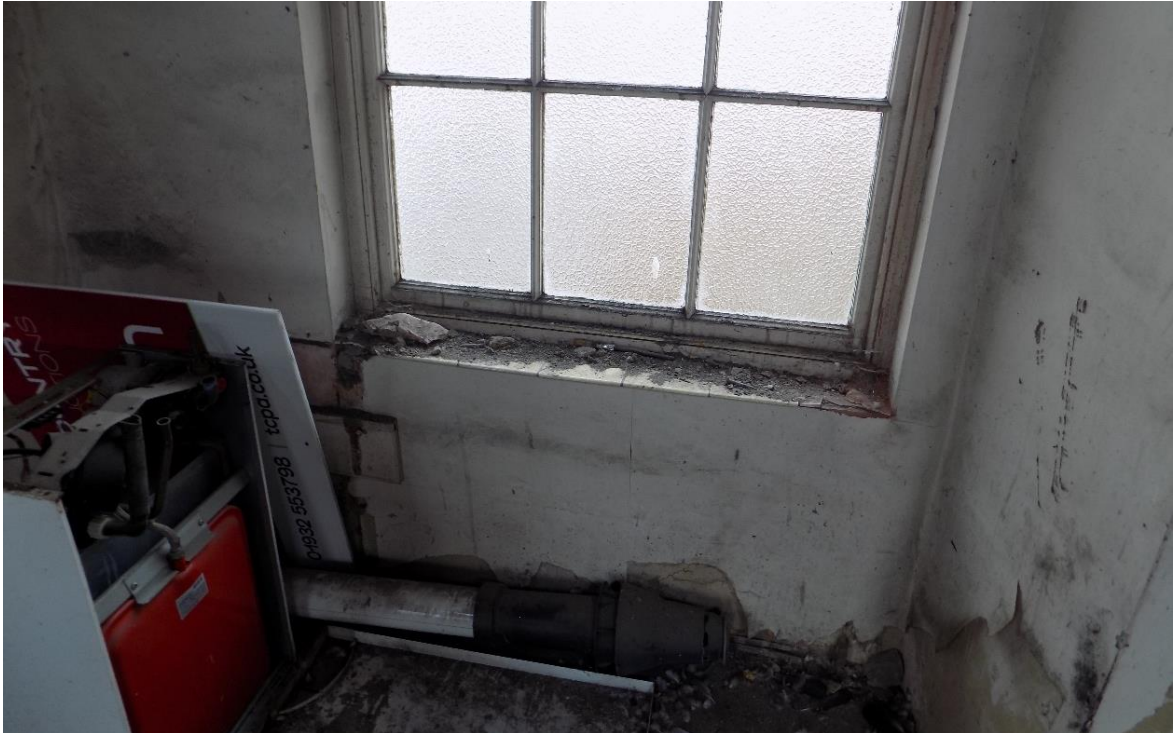
Fig.30: First-floor: Detail of first rear-facing window from west, showing ten-inch wall below and to left.
