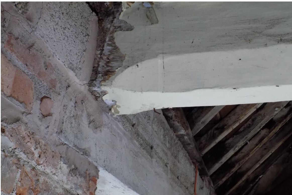
Fig.42: Detail of chamfers and curved step stops to the first and second trusses from the east.
