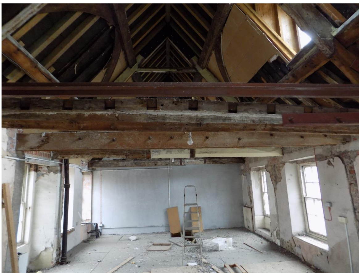
Fig.37: General view of roof, showing truss ties and beam flitched with modern softwood.
