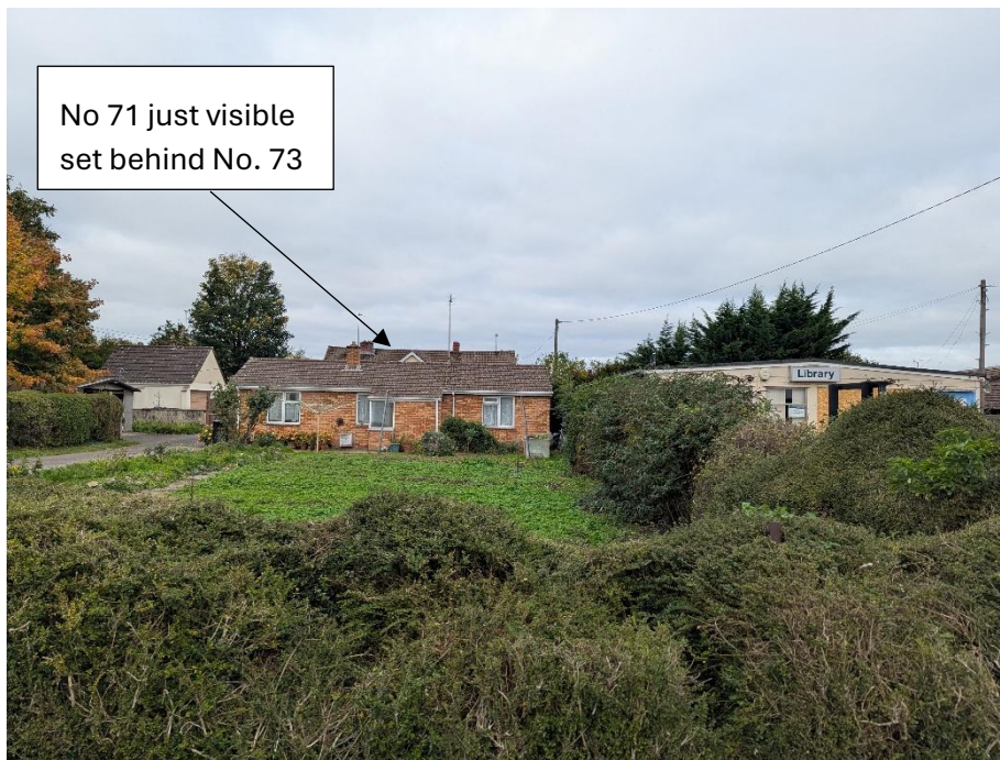
Figure 10 - No.71 when viewed from the pavement outside the appeal site
