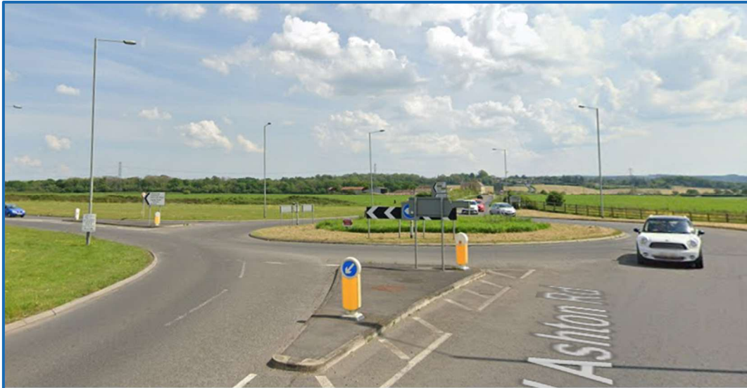
Figure 5 - Existing Lighting on the roundabout of West Ashton Road and Leap Gate (Google Maps, May 2024)
