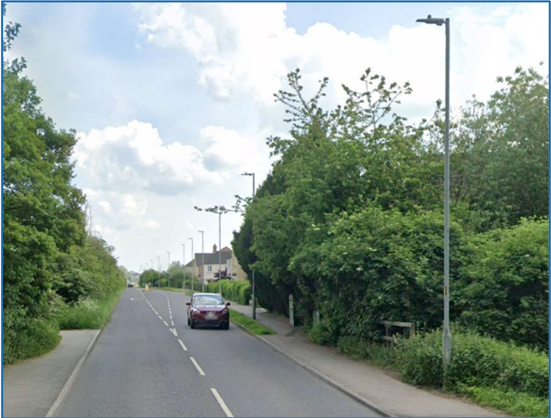
Figure 4 - Existing Lighting along West Ashton Road
