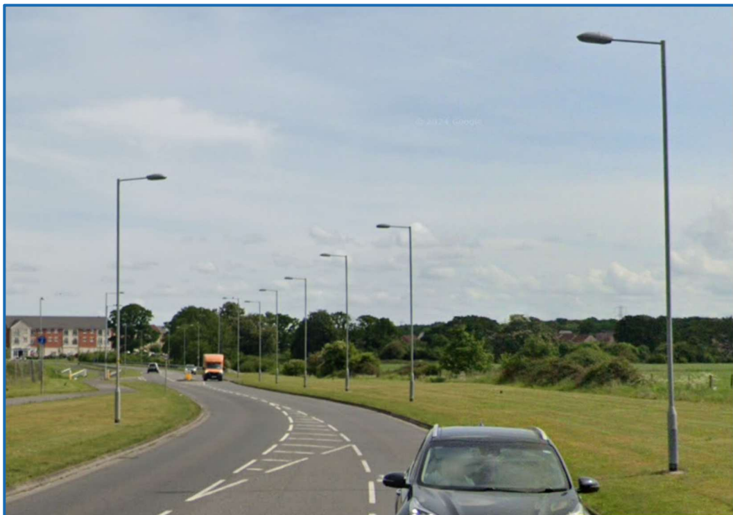
Figure 6 - Existing streetlighting along Leap Gate (Google Maps, May 2024)
