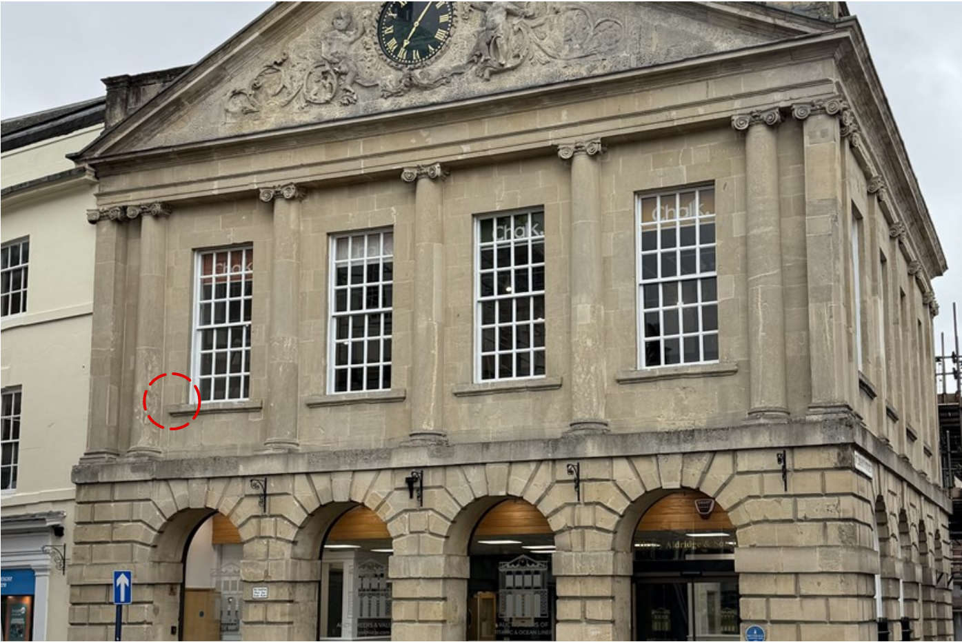
Figure 1: Location of cable on external north facade (imperceivable from street)
