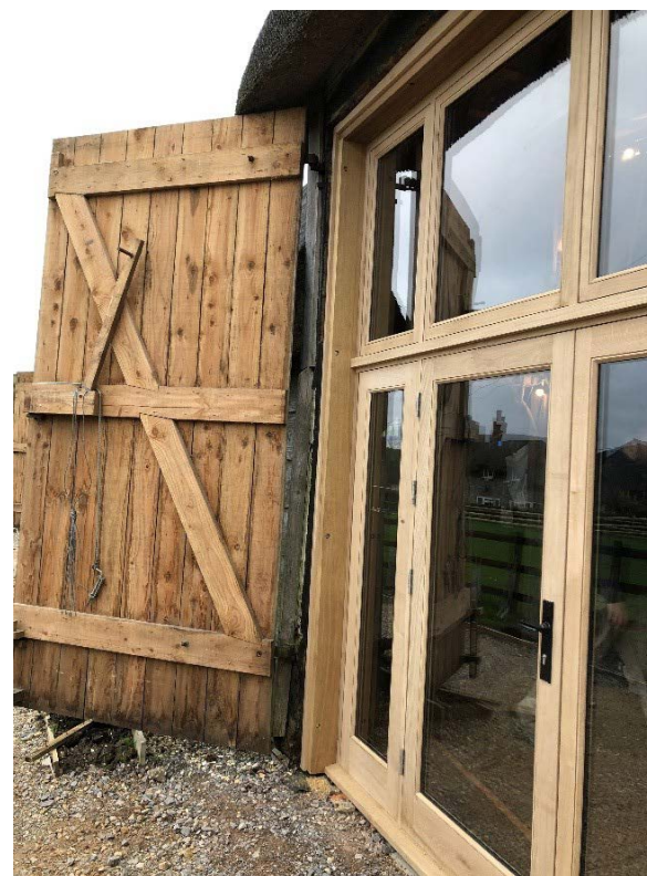
Fig. 9 - Photograph shows the recently installed glazed oak joinery
