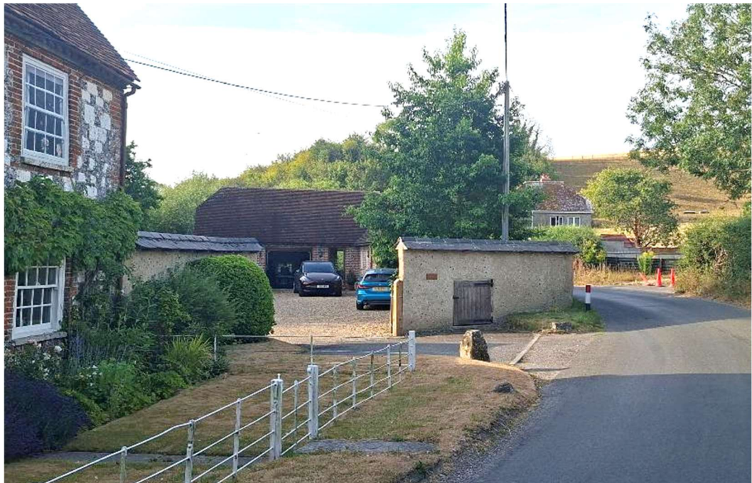
Figure 12 From opposite Woodford Mill looking south, a private house adjacent to the former local authority houses can be seen, the relationship shows that whilst the density of development may be lower than in the core of the village, the mill is clearly part of Middle Woodford. The modern garage and pool building to the mill is also seen in this view.
