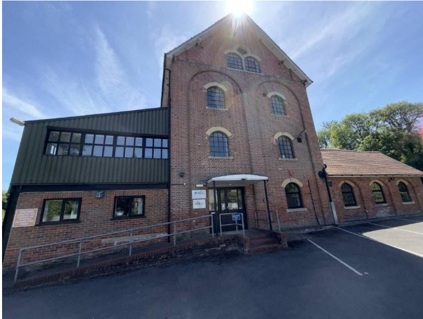
Photograph 01 Boreham Mill, Bishopstrow Road, Warminster, BA12 9HQ
