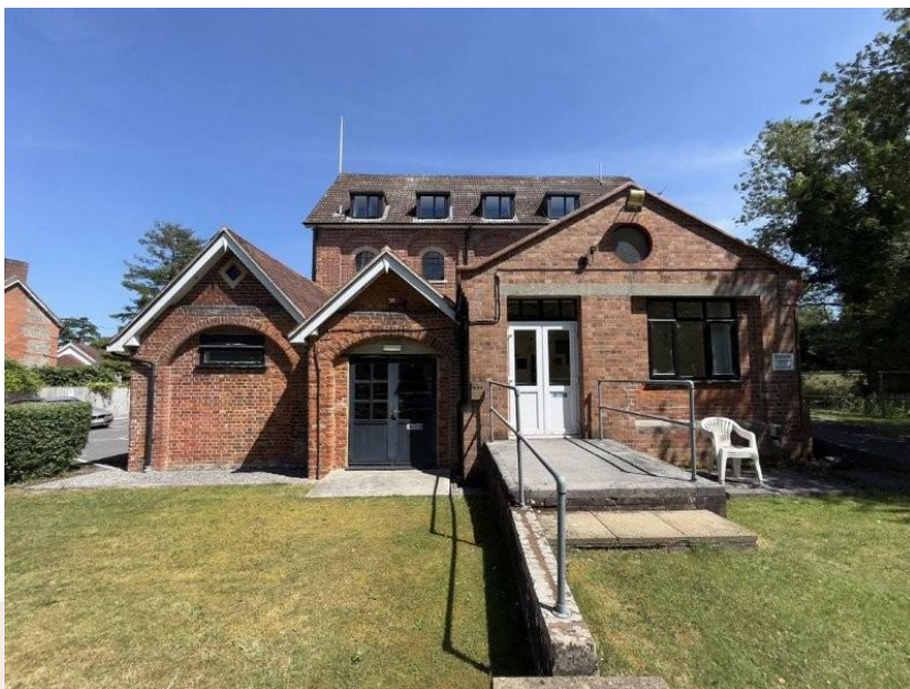
Photograph 02 Boreham Mill, Bishopstrow Road, Warminster, BA12 9HQ
