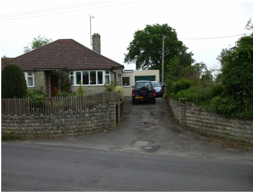
No 19 Ball Road original bungalow with small garage in 2008 seen from Ball Road with wall, shrubs and bushes hiding views to open land to the east.
