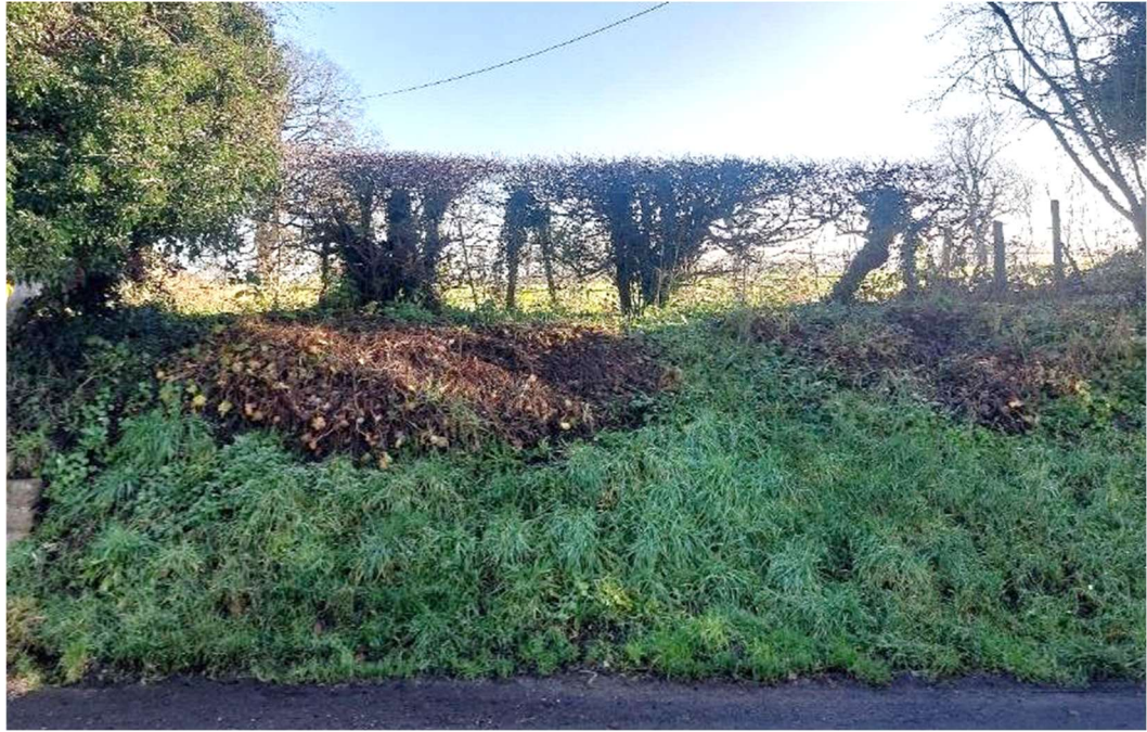
Figure 4 The proposed development site from the immediately adjacent section of Ball Road, looking east.
