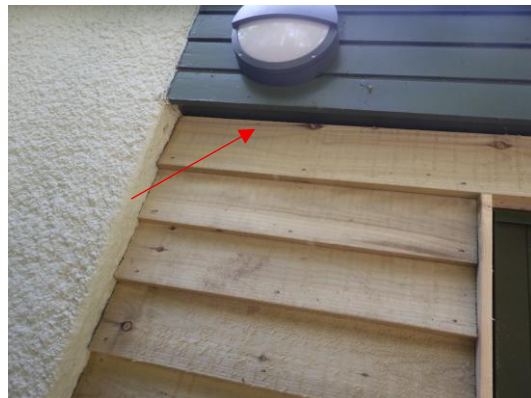
Example of a potential roosting / nesting feature which is present due to the natural gaps created within timber during construction (image taken from a different project at a different Center Parcs village)
