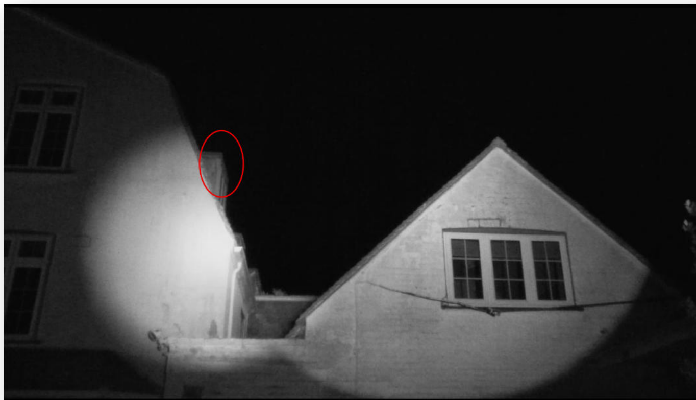
Figure 10. Screenshot of camera footage showing the potential bat egress locations on the southwest elevation of B1
