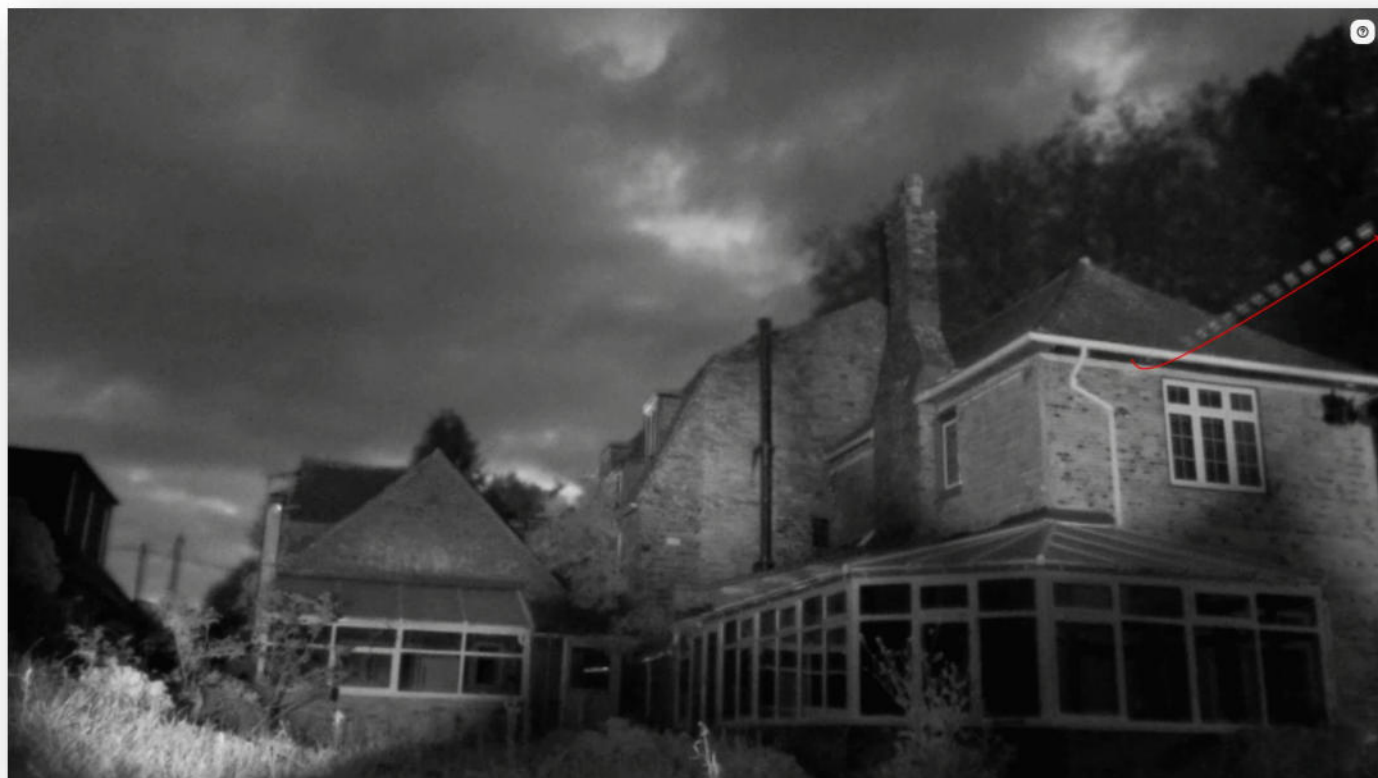
Figure 14. Image showing the emergence of a serotine from the southeast elevation of B1 on 05/05/2026 at 21:23
