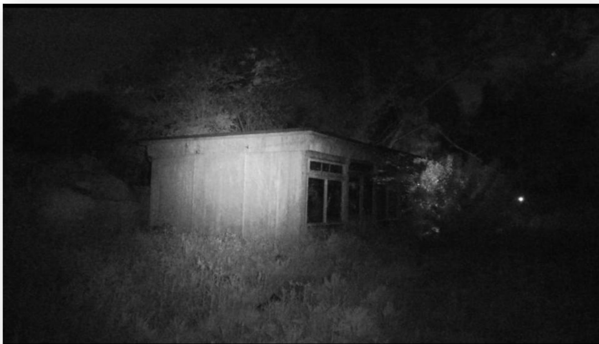
Figure 6. Screenshot of camera footage showing the northwest elevation of B3
