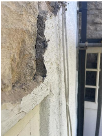
Cementitious render applied to front elevation
