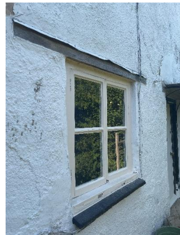
Existing opening with timber lintel
