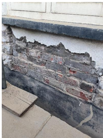
Modern brickwork repair to front elevation.
