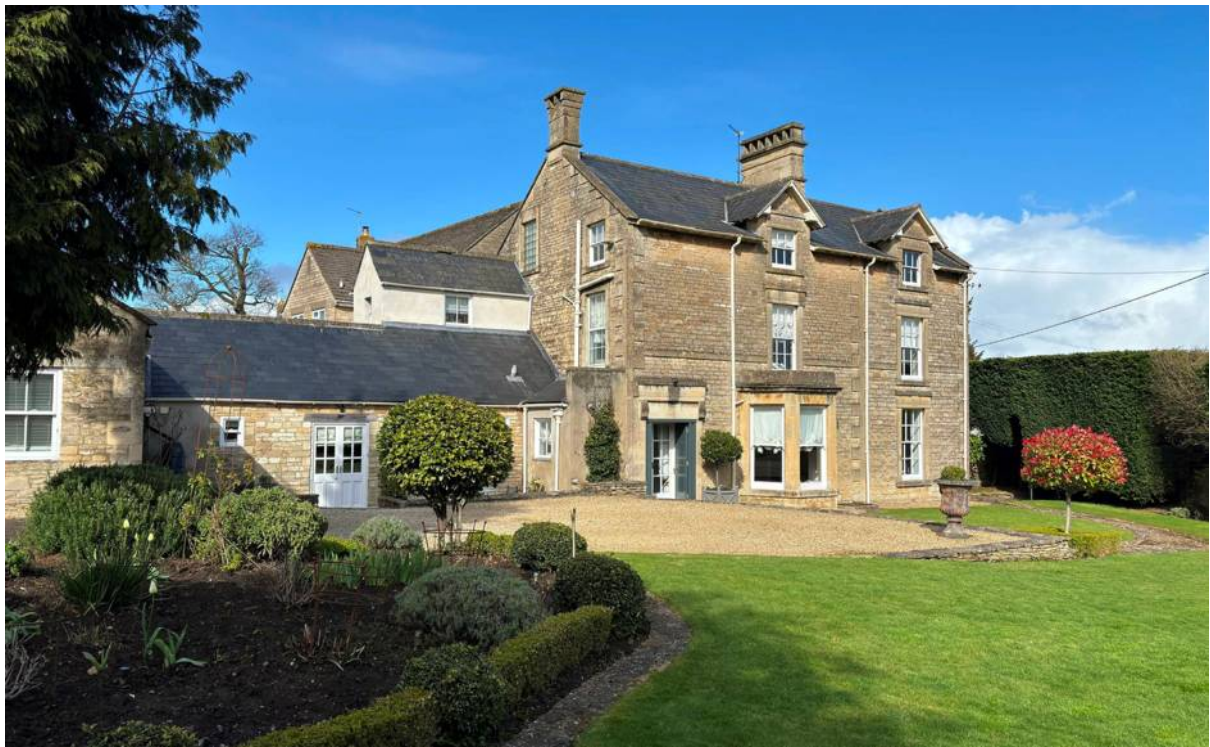
Existing site photograph
