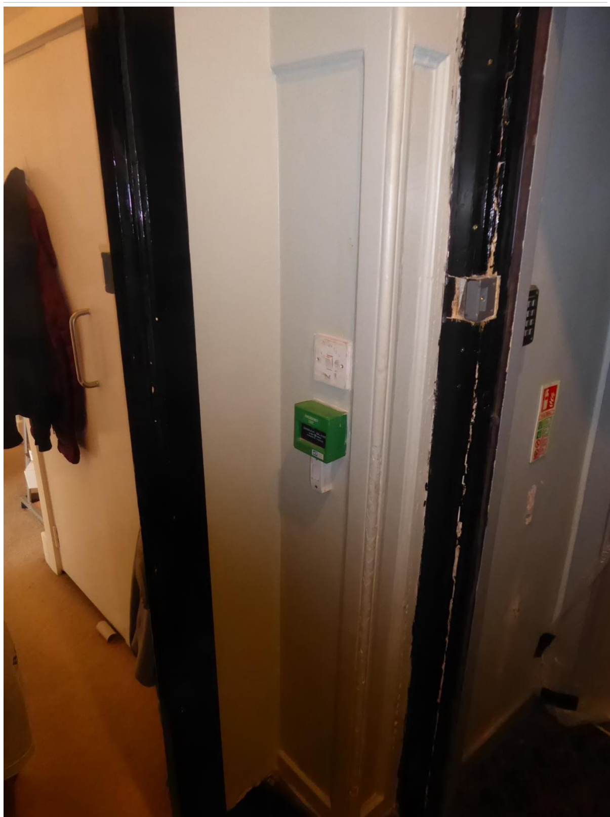
Figure 16: Decorative arch in 'caretakers flat' partially exposed
