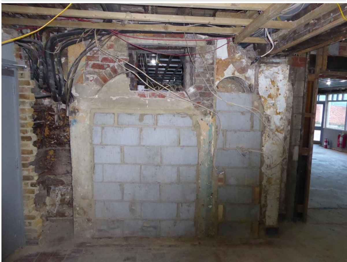
Figure 13: Potential former fireplace (later opening) with niches – back wall of former hotel (prior to modern extension) – area referred to as ‘Old Kitchen’ in 1929 plans (see Appendix I )
