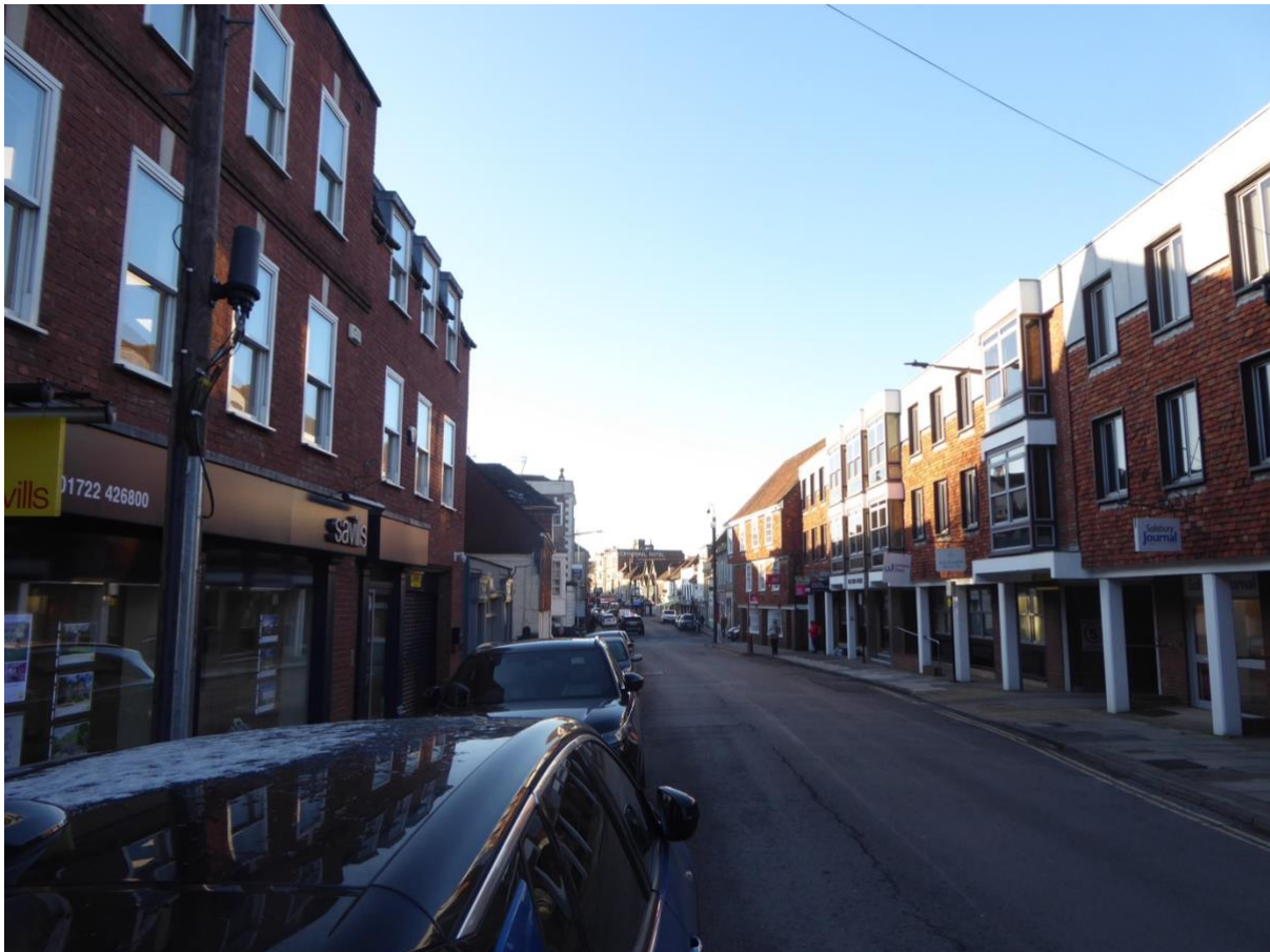
Figure 4: View of east elevation of Cathedral Hotel from Milford Street/Hill
