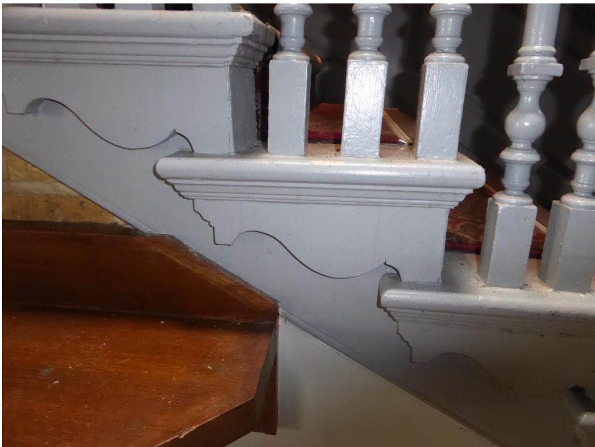
Figure 9: Decorative brackets to each tread of 18 th century stair
