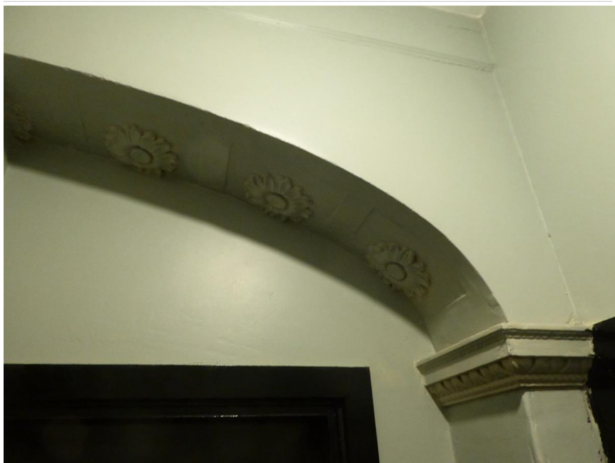
Figure 15: Decorative arch in 'caretakers flat' partially exposed
