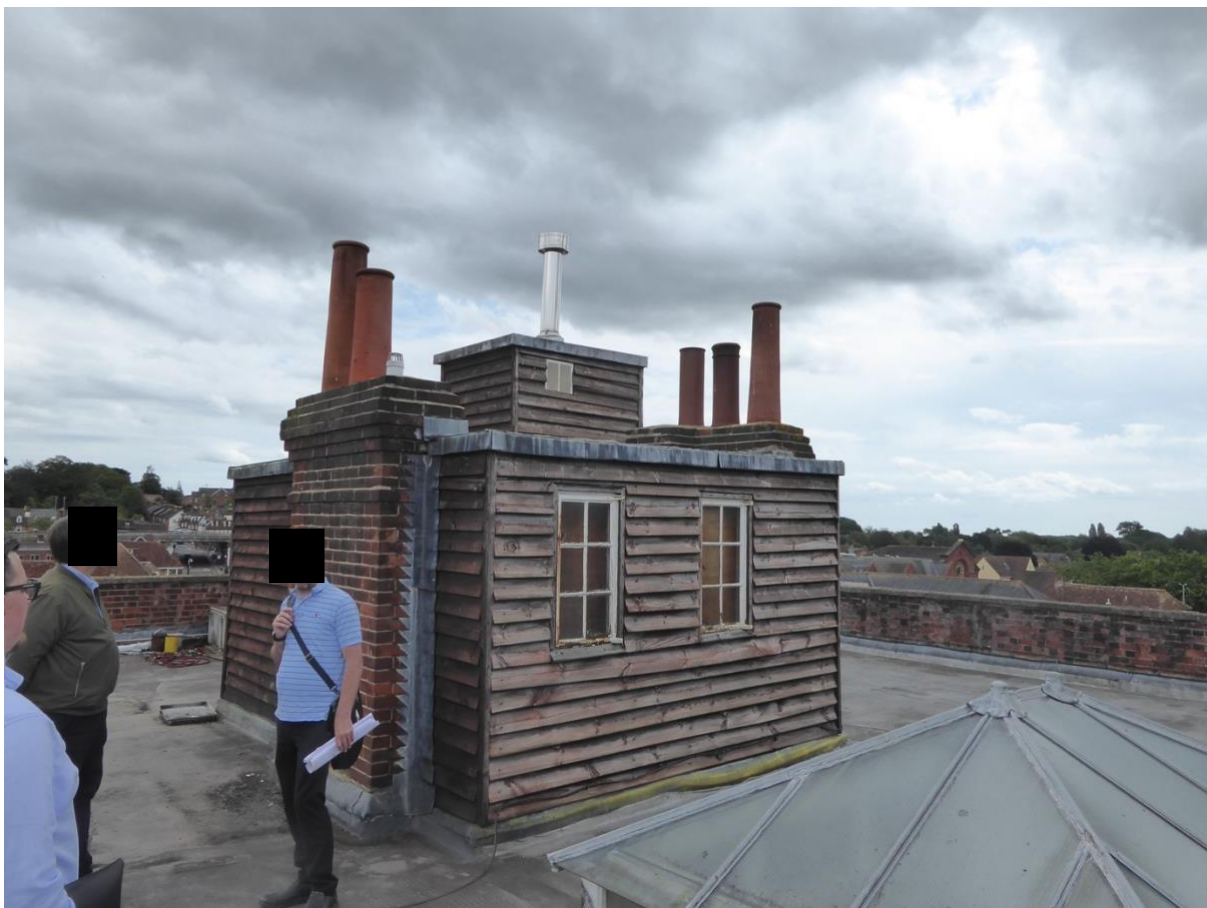
Figure 6: Plant room and stair access to roof between brick chimneystacks
