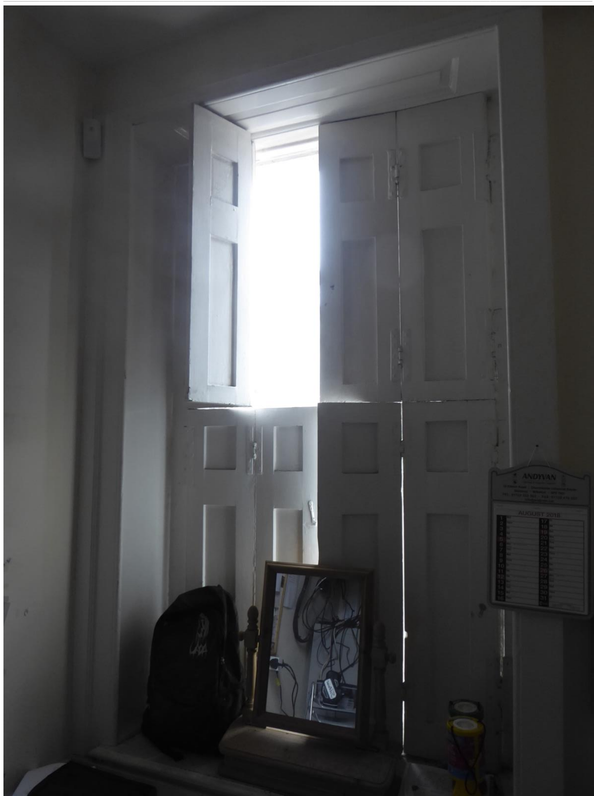
Figure 17: Panelled shutters to earlier window in south elevation (presently in 'caretakers flat')
