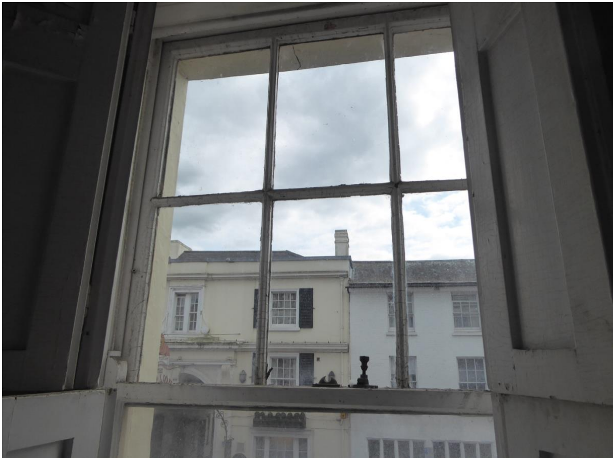
Figure 21: Older sash to window in front elevation (probably early to mid 19 th century)
