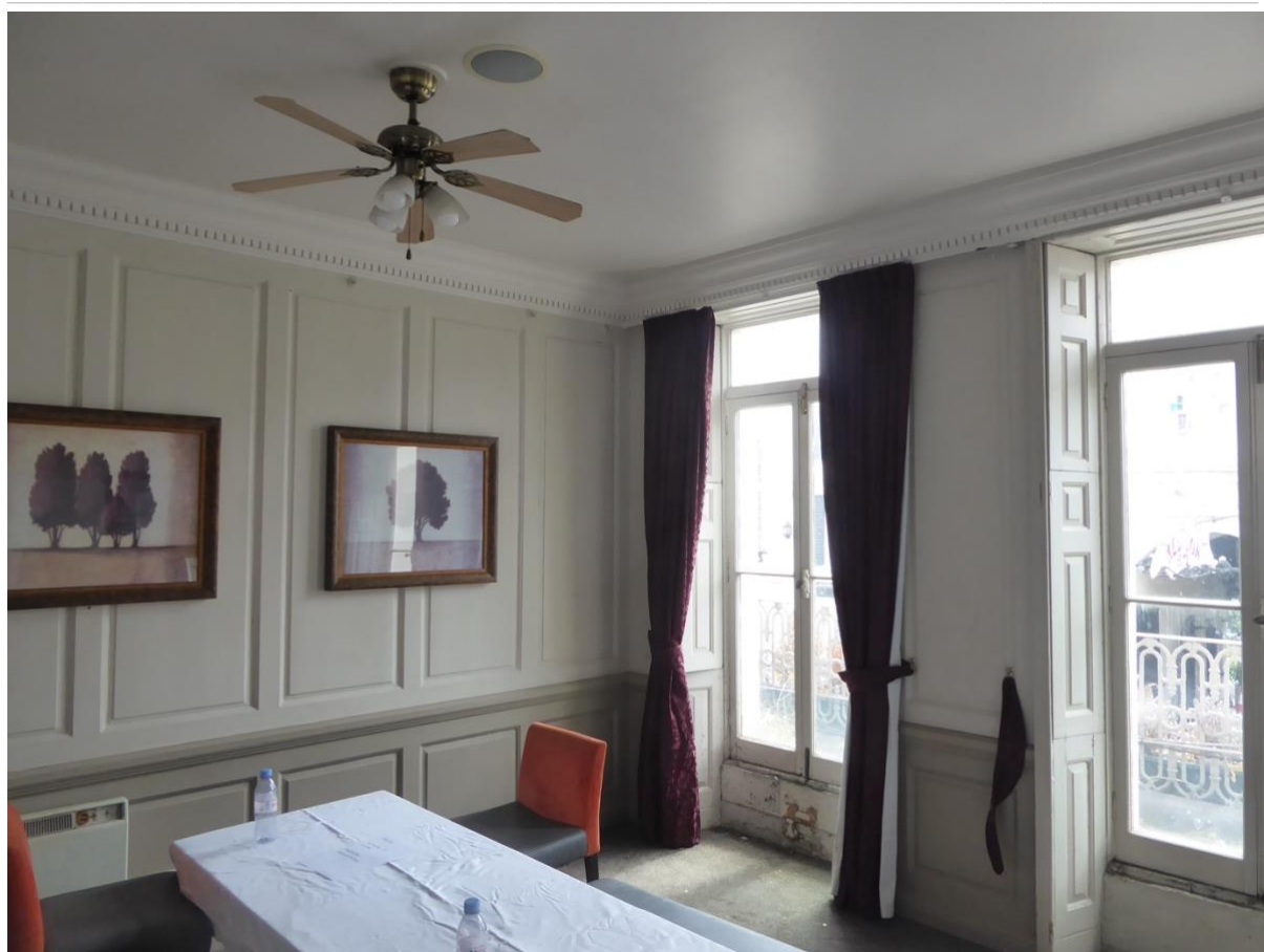
Figure 14: Panelled room to first floor front (centre) with cast iron balcony
