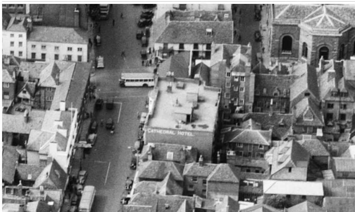
Figure 3: Extract from Historic England EAW051918 ENGLAND (1953) New Canal, the Market Place and the city centre, Salisbury 1953 – Cathedral Hotel east elevation and buildings to rear
