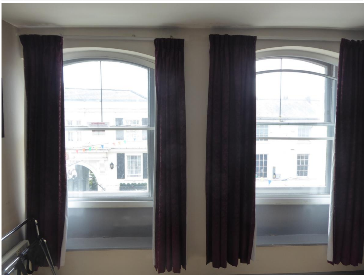
Figure 19: Typical vertical sliding sashes with vertical 'glazing' steel bar to top sash
