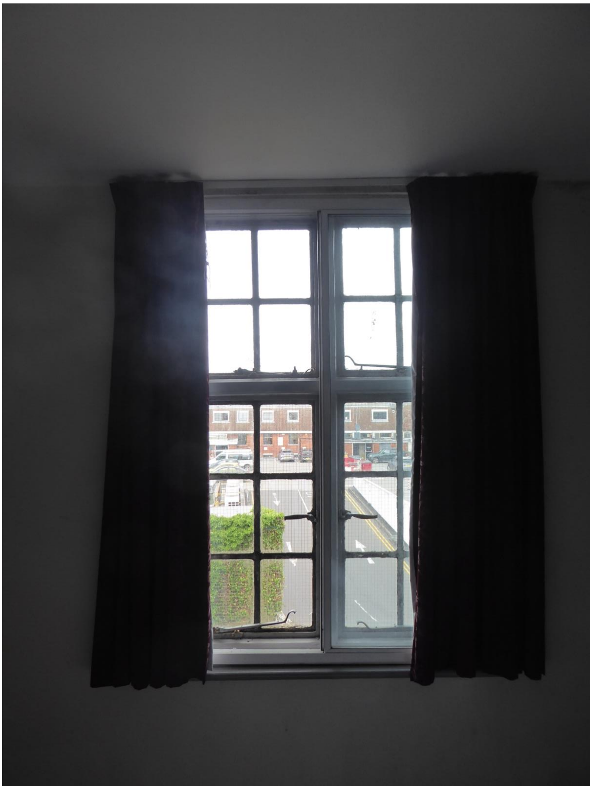
Figure 22: Typical metal casement windows to rear elevation (post 1929 alterations)
