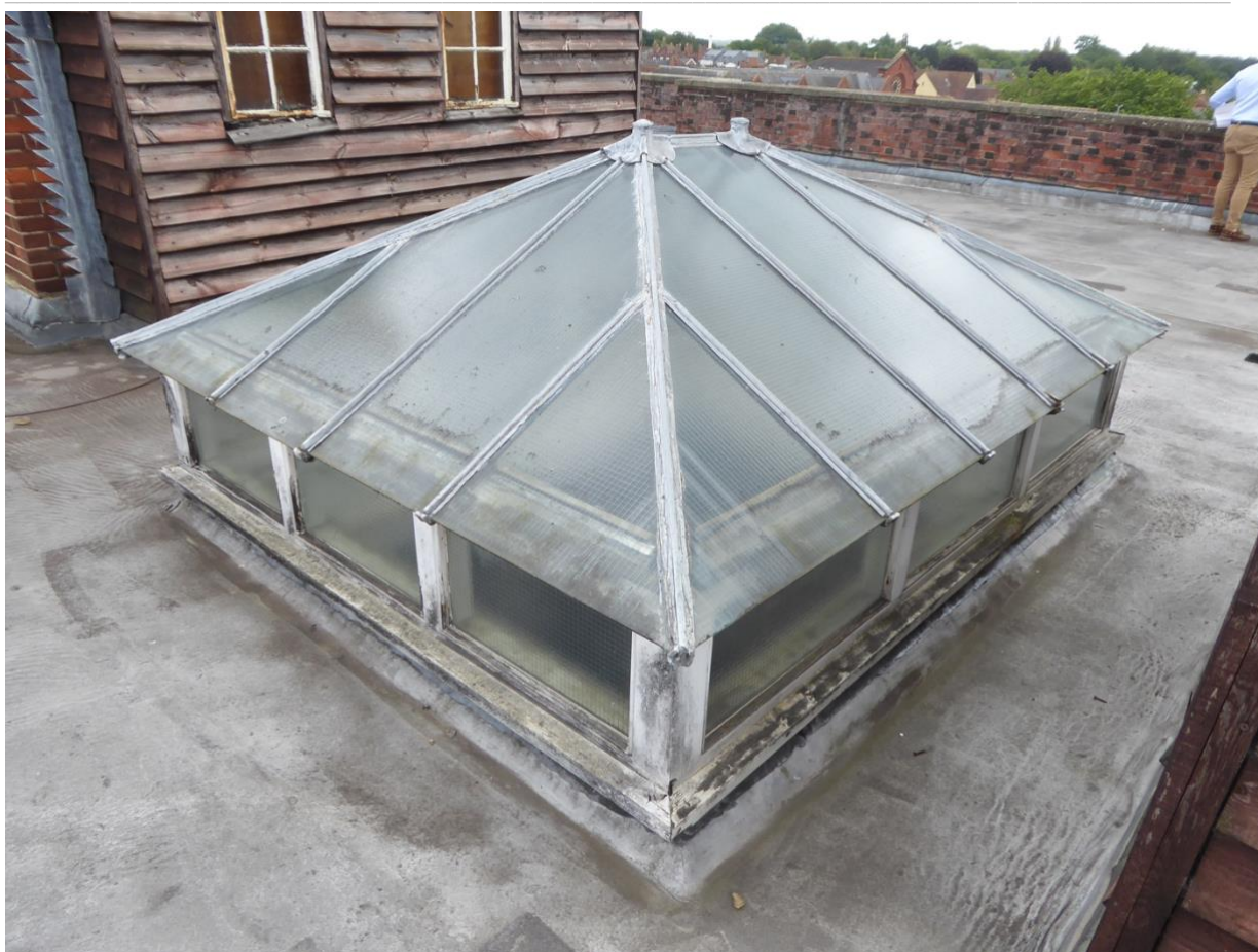
Figure 26: Modern roof lantern above staircase
