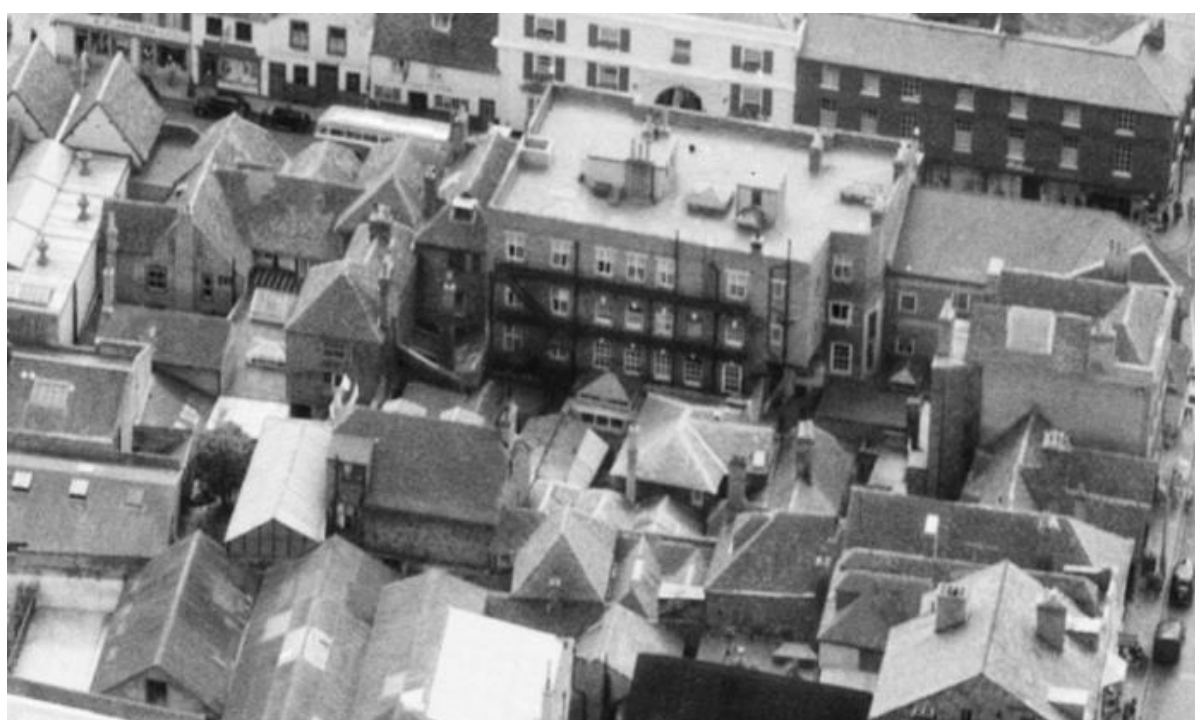
Figure 4: Extract from Historic England EAW051919 ENGLAND (1953) Brown St, the Guildhall and the city centre, Salisbury 1953 – Cathedral Hotel north elevation and buildings to rear
