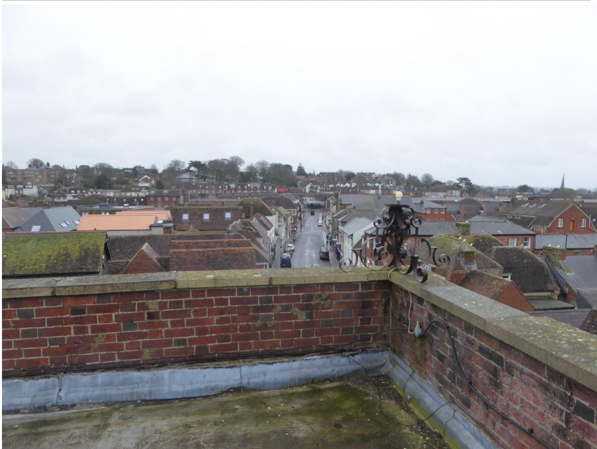
Figure 5: Modern decorative light fittings to corners of hotel on parapet
