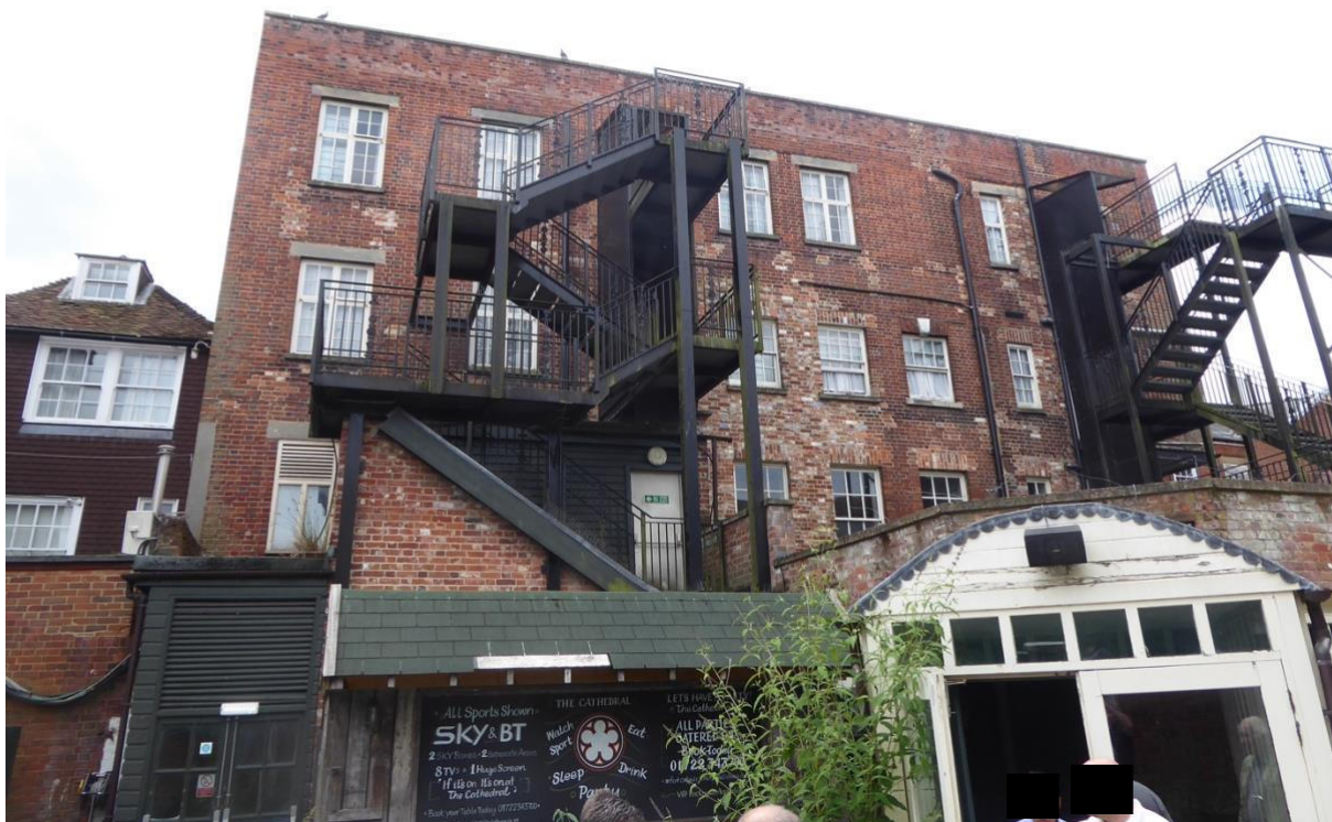
Figure 2: North/rear elevation Cathedral Hotel
