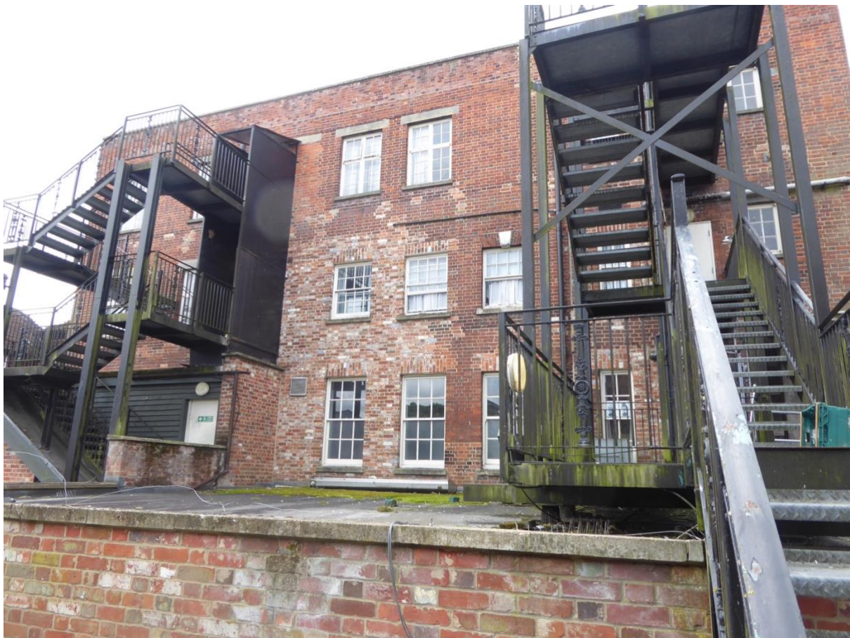
Figure 3: Older windows to central section of rear elevation
