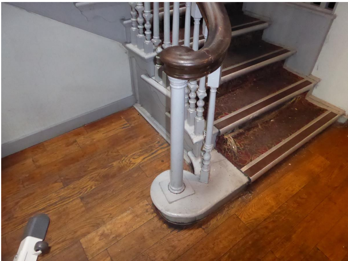
Figure 10: Detail of curtail step to 18 th century stair
