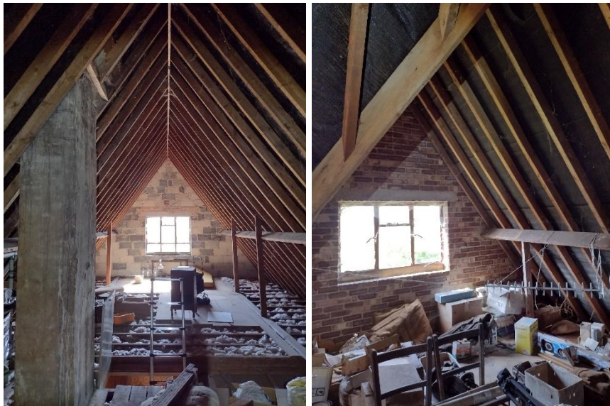
Figures 14 and 15: Eastern and southern section of the roof void
