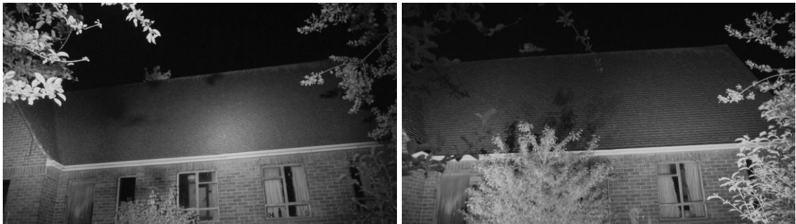
Figure 1 and 2: Still from Infra-Red camera facing southeastern elevation in 2024 and 2026
