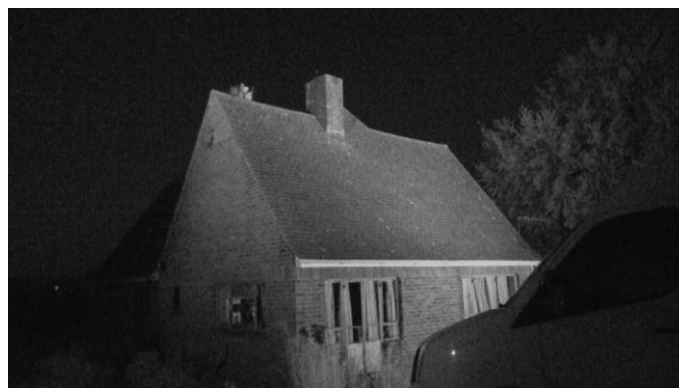
Figure 5: Still from Infra-Red camera facing western elevation in 2026
