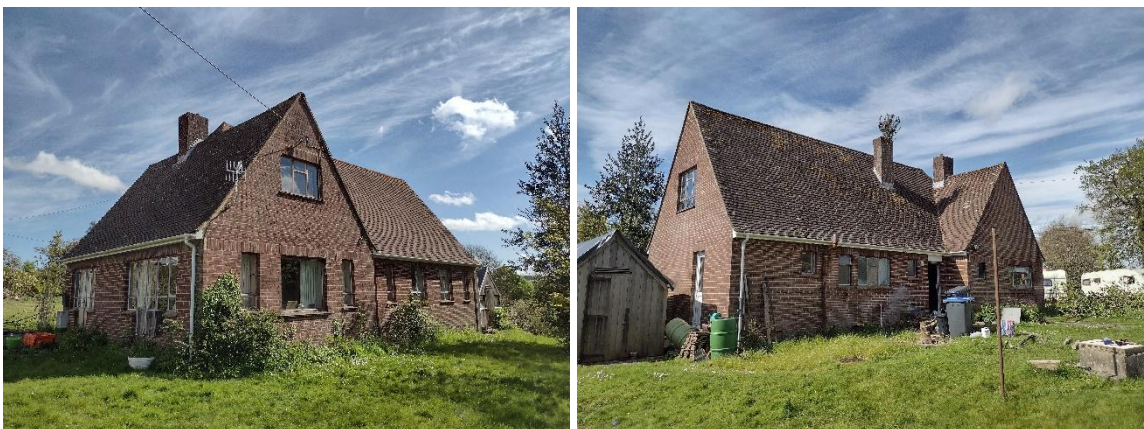
Figures 12 and 13: Residential building.
