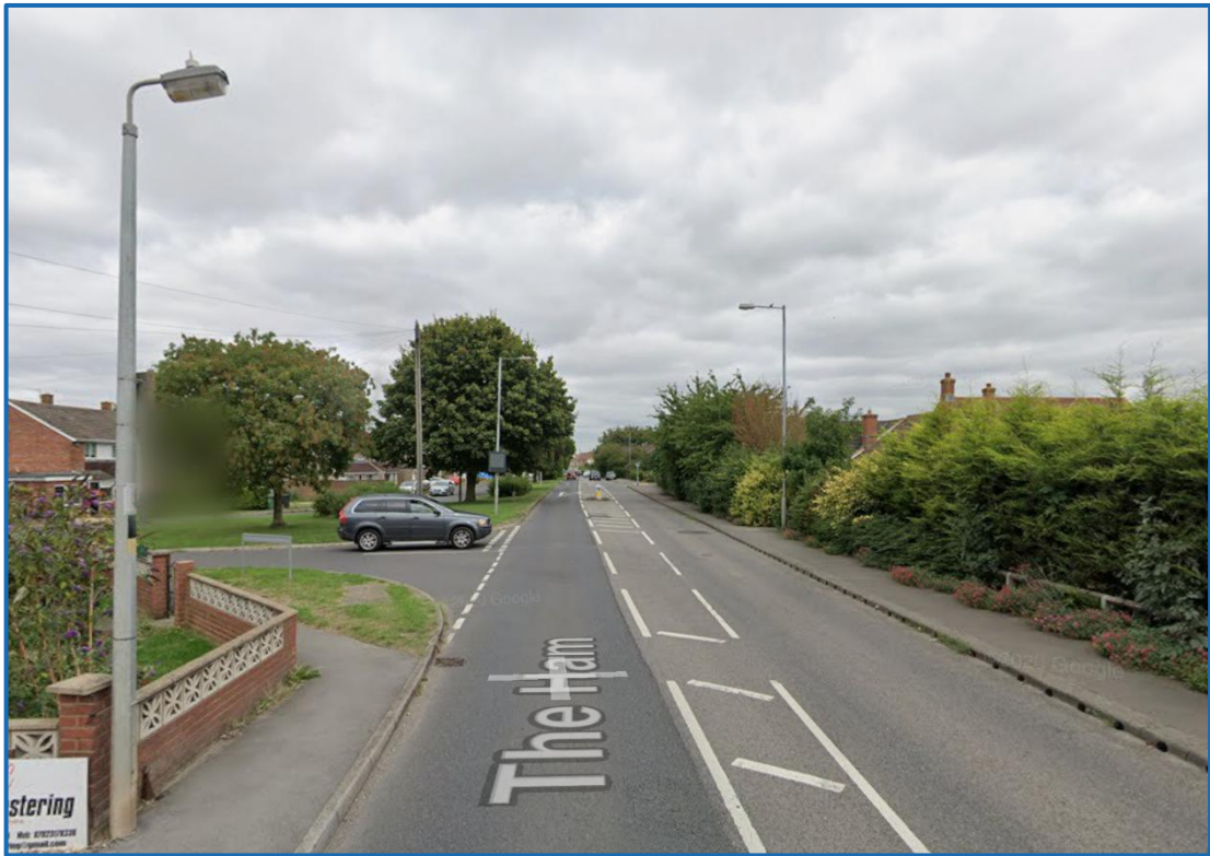
Figure 9: View of the existing street lighting from The Ham
