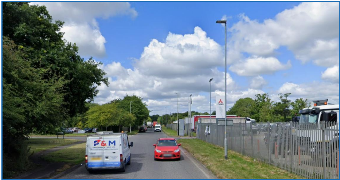
Figure 5: View of existing lighting from Broadway N road
