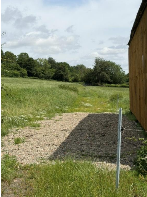
Left: Rear (north west) elevation of the barn with access track to the left leading to Tutton Hill.
