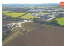
Aerial view of site area for proposed commercial space
