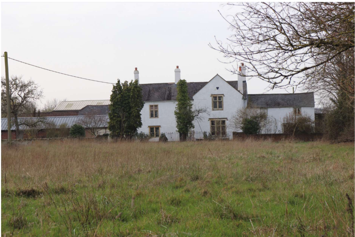
Plate 8 The best view [3] of the farmhouse from the field to the east which lies outside the Application Site, viewed from the public right of way
