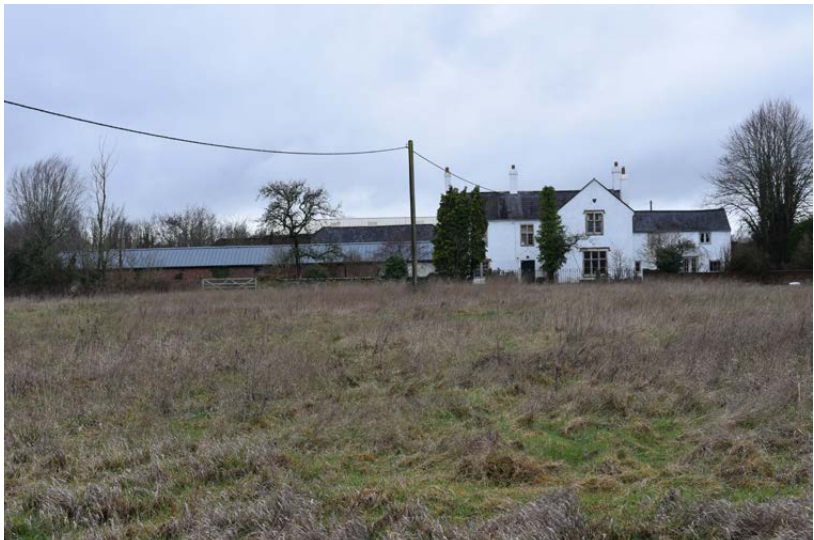
The Grade II Listed Hawkeridge Farmhouse is seen via glimpsed views through the vegetation in various places across the site and seen in it's entirety from the off Site PRoW connecting the two parcels.
