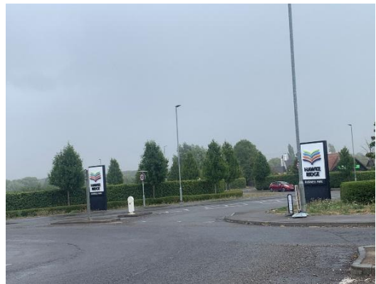
Photo 13 Developed land; sealed surface habitat in east of site (A15)
