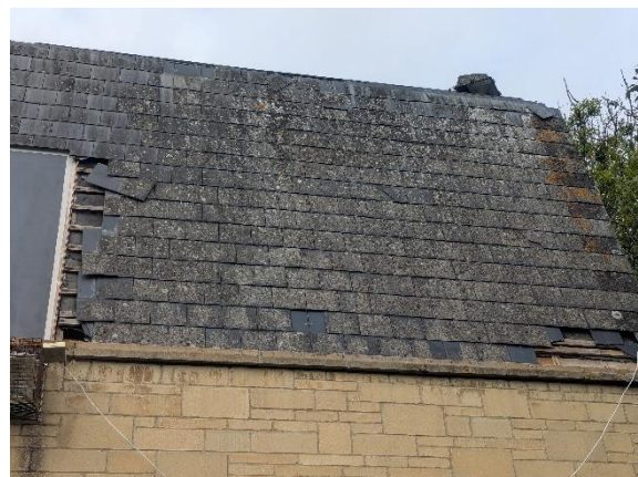
Photo 6 – external view of broken and slipped tiles
