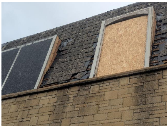
Photo 5 – external view of slipped and broken tiles
