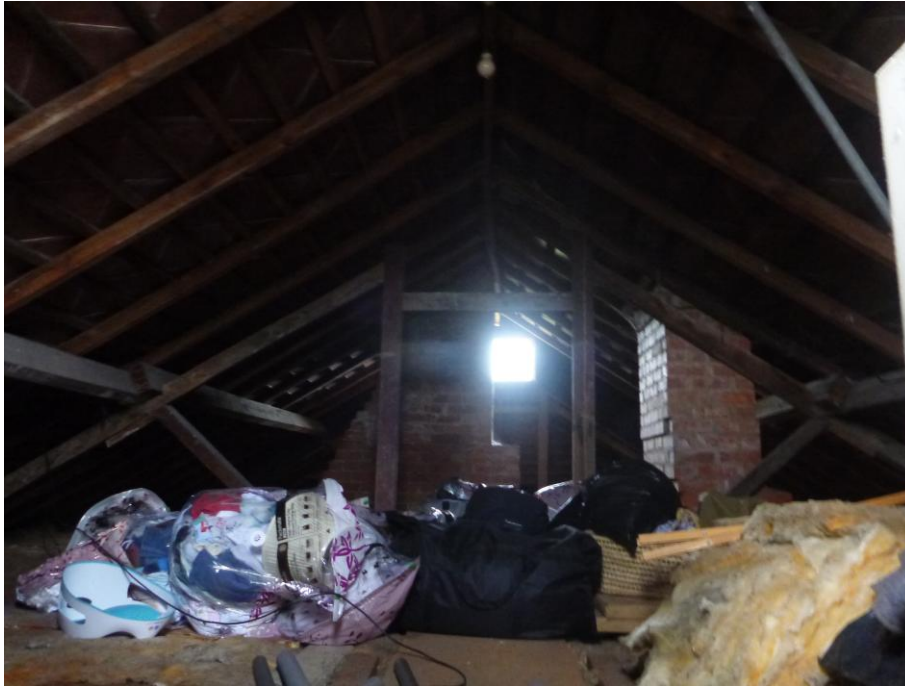
Fig 6: Windows in the gable ends allow daylight to penetrate the loft space.
