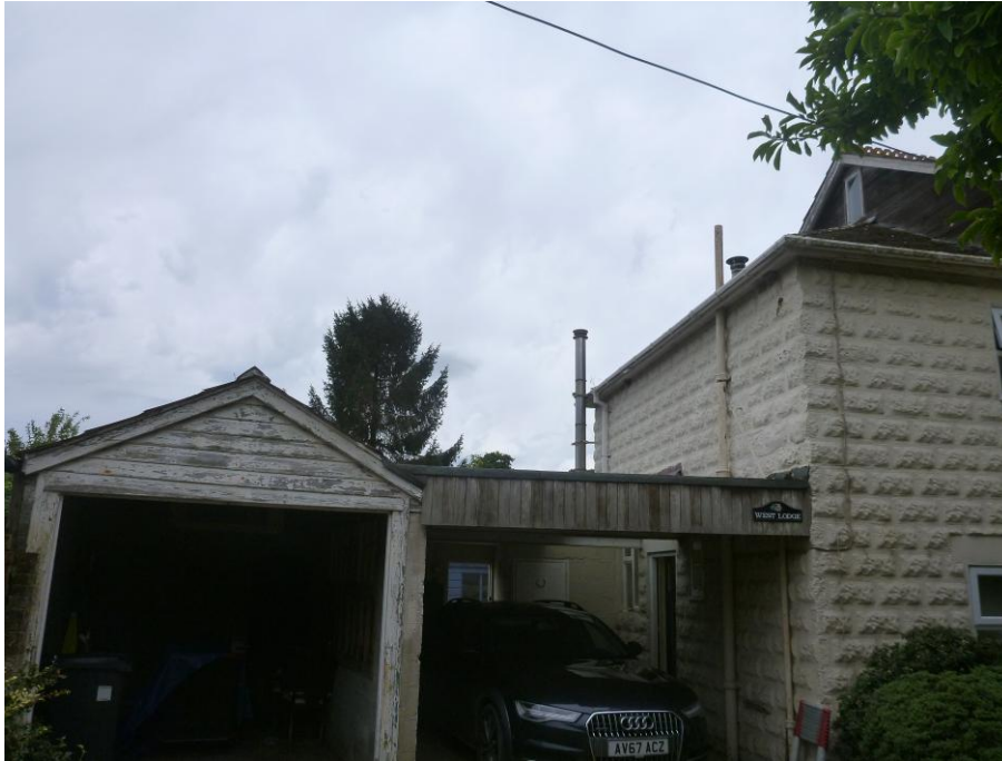
Fig 4: Single storey garage and car part attached to the east face of West Lodge.
