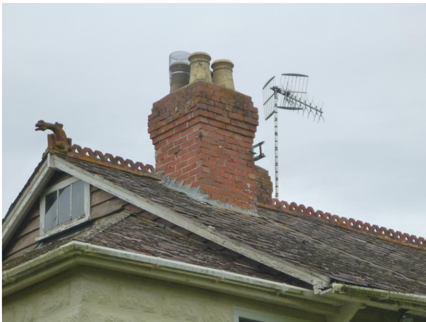
Fig 3: A lower roof ties in on the western gable which is clad with timber.
