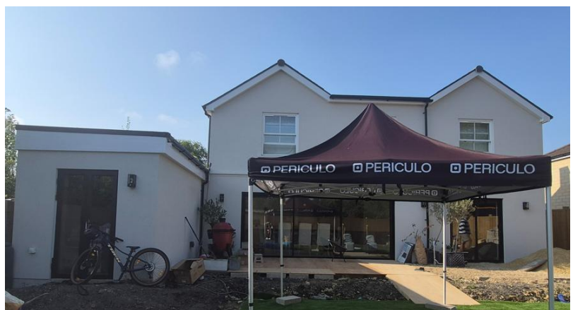
(L-R) Existing Front and Rear of the Dwelling
