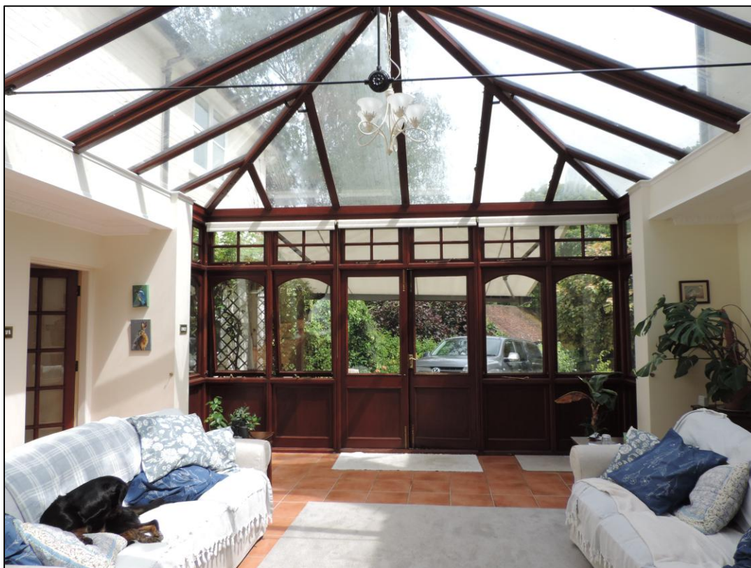
Photo 2 North-east facing view within the 1995 conservatory style link. Photograph date 16th June 2026.
