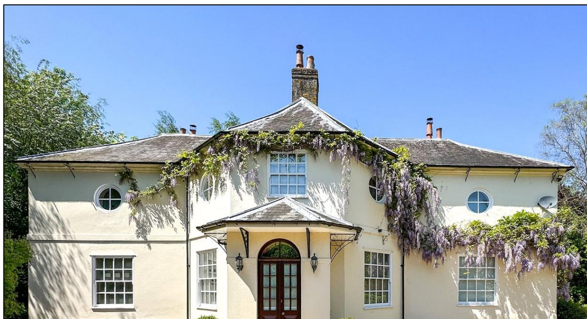
Figure 3 Principal south-east facing elevation Manor Farm. Source https://www.fineandcountry.co.uk
