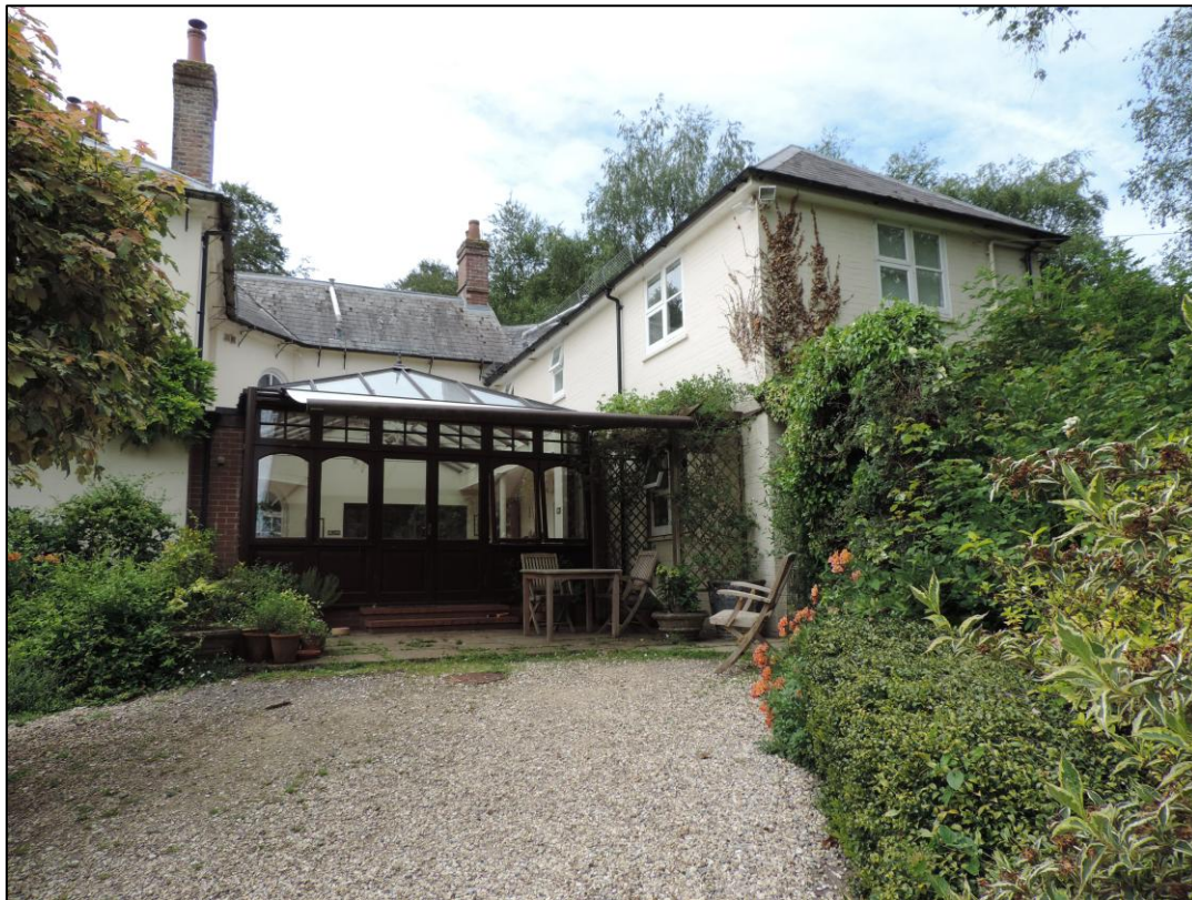
Photo 1 1995 conservatory link between the 1830s core and 1995 extension. West facing view.
