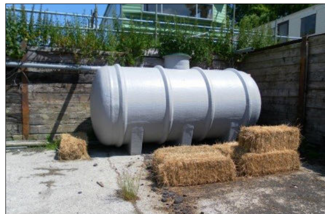
Sample accommodation units and waste storage tank located in former silage clamp.
