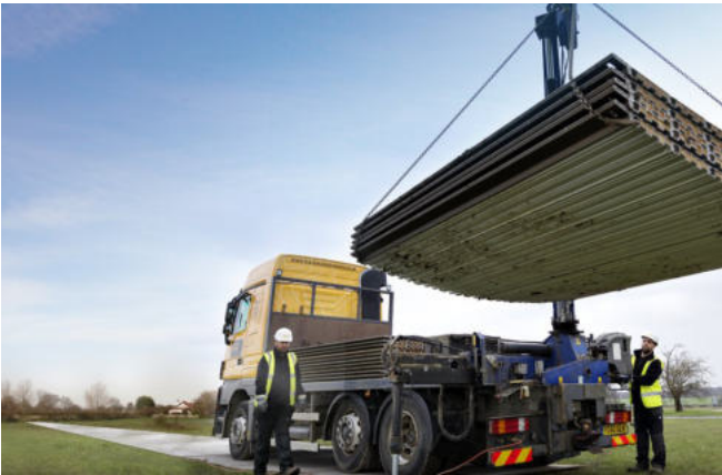
Above. Sample images showing temporary sheeting material for parking and access tracks.
