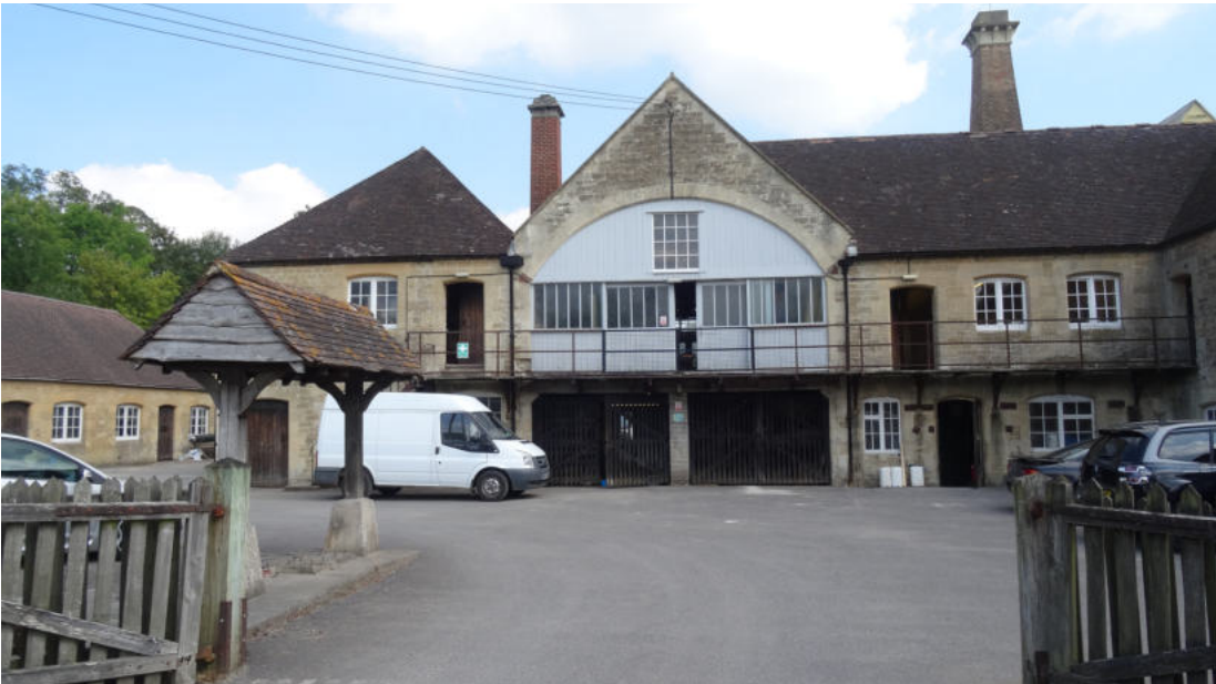
Photo 1 Stalls Farm. Front of main office / administration building from Estate boundary roadway.
