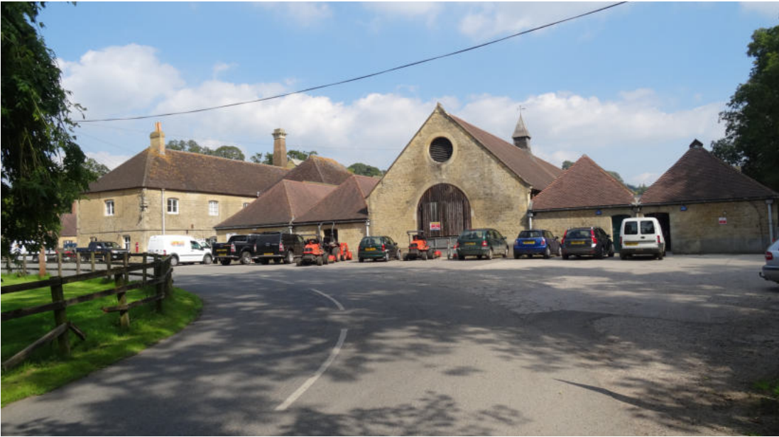
Photo 2 Stalls Farm. Front of storage buildings from Estate boundary roadway.
