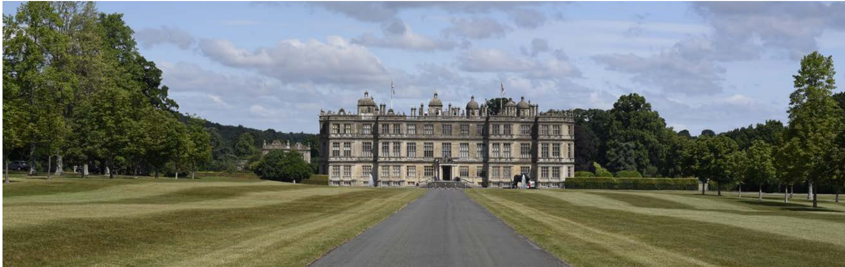
View 1: View from Horningsham Drive by day
