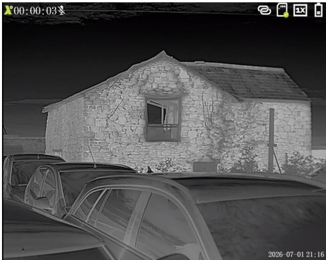
Photograph 1: - Western aspect of building B1 - IR image at start of survey – 01.07.26
