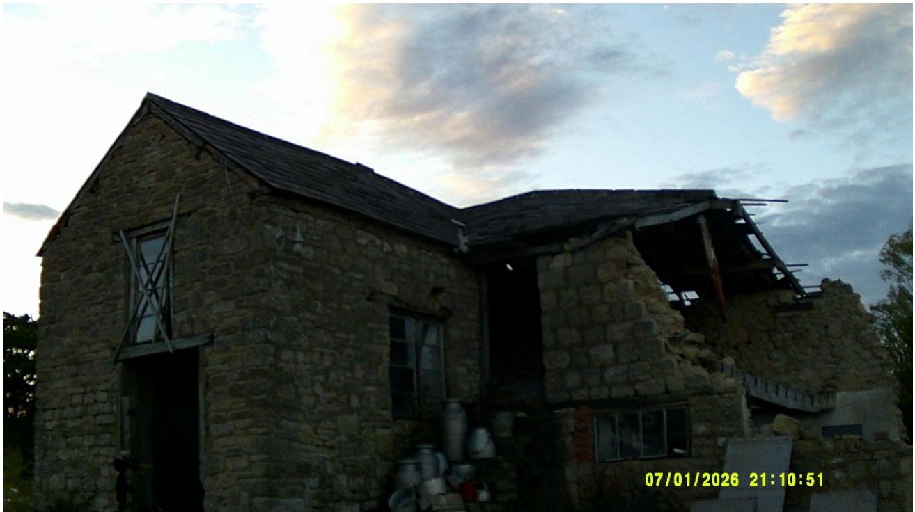
Photograph 4: Eastern aspect of building B1 - IR image at start of survey – 01.07.26
