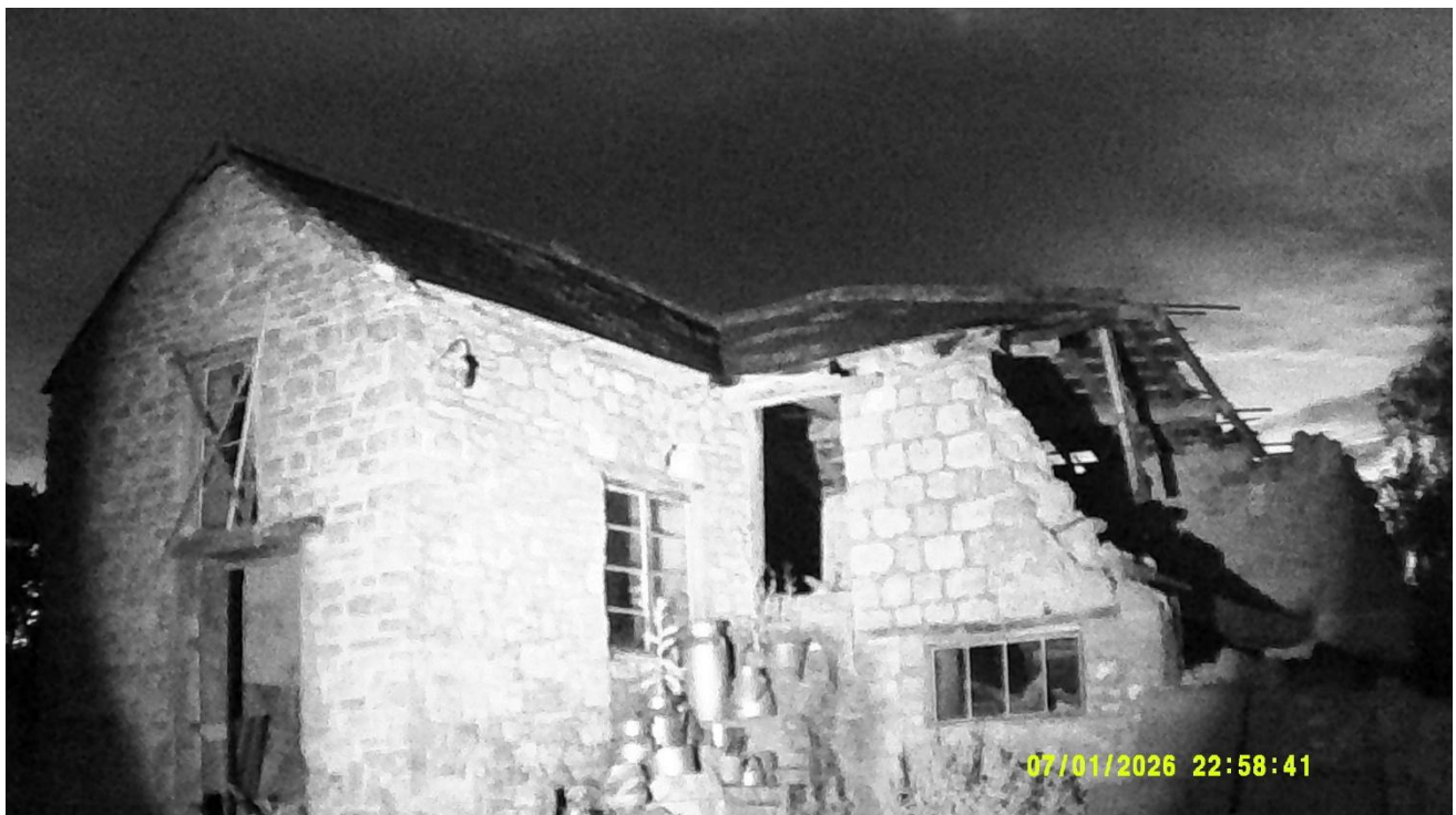
Photograph 4: Eastern aspect of building B1 - IR image at end of survey – 01.07.26
