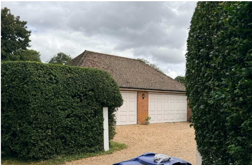
West Stowell Walk Tiled hipped roof garage
