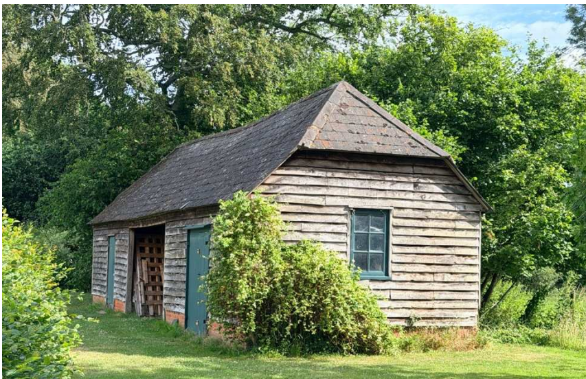
Storage Barn West Stowell Estate Slate hipped roof outbuilding
