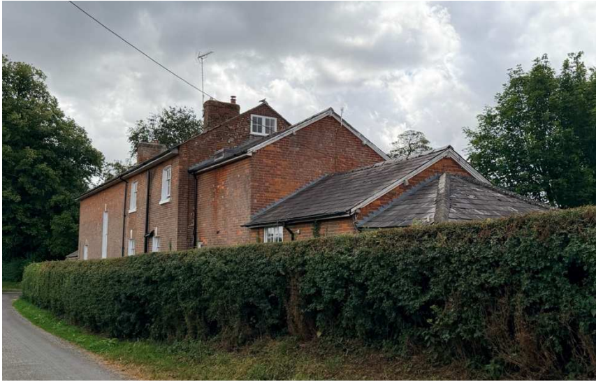
West Stowell Farmhouse Natural slate roof finish
