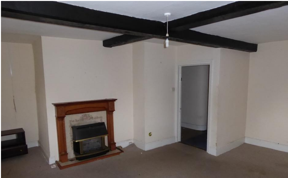
Figure 20: Room above kitchen with 17 th century beams
