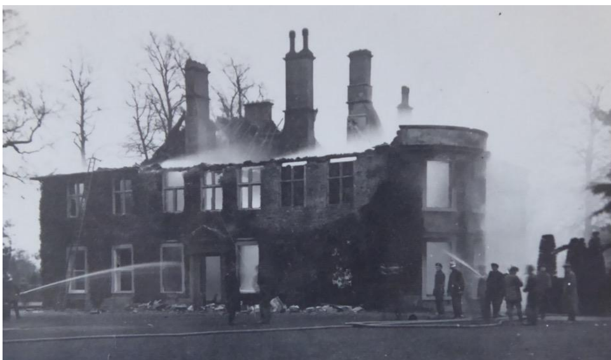
Figure C4: Melksham House 1920; immediate post-fire north elevation
