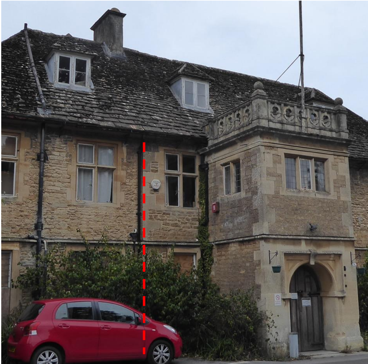
Figure 7: North section, east elevation – straight joint defined by quoins
