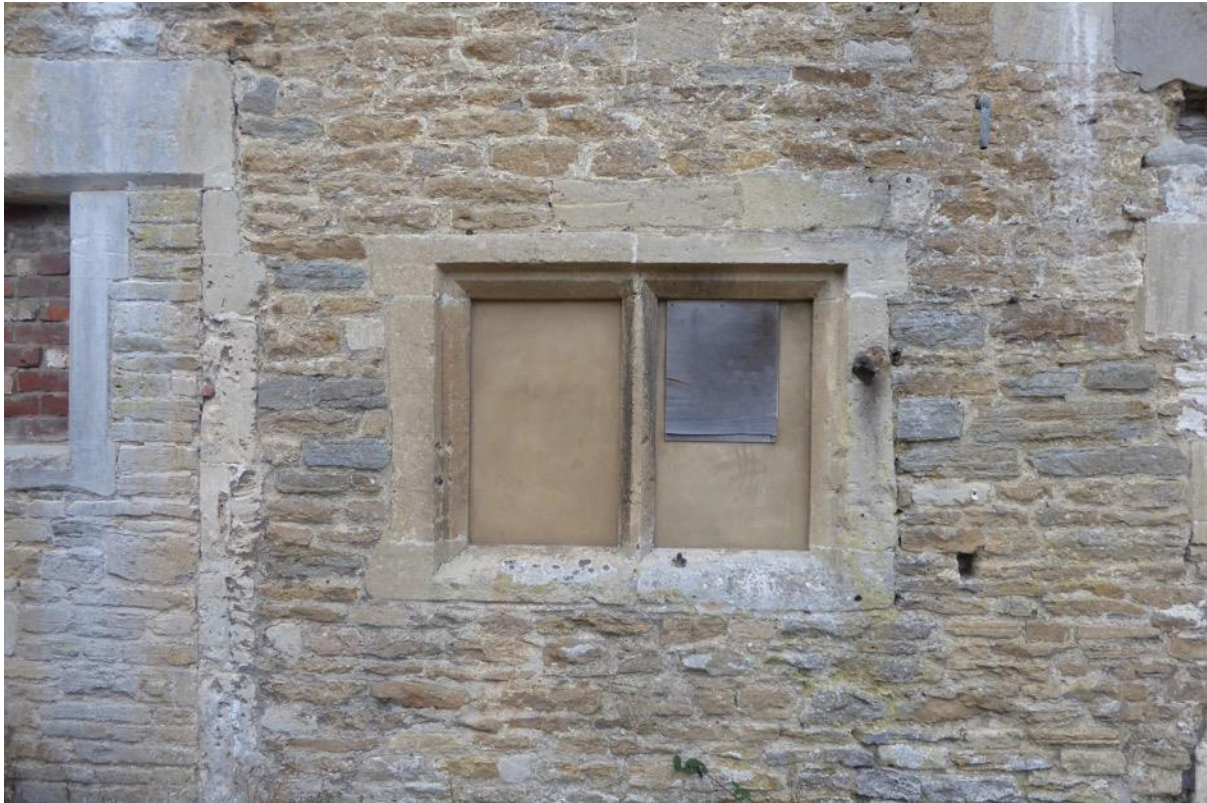
Figure 33: Stable block, possible re-used 17 th century window (now blocked)
