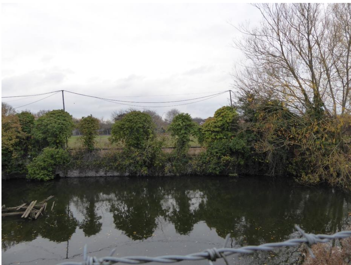
Figure 42: Ornamental pond (from north) with rubble stone retaining walls
