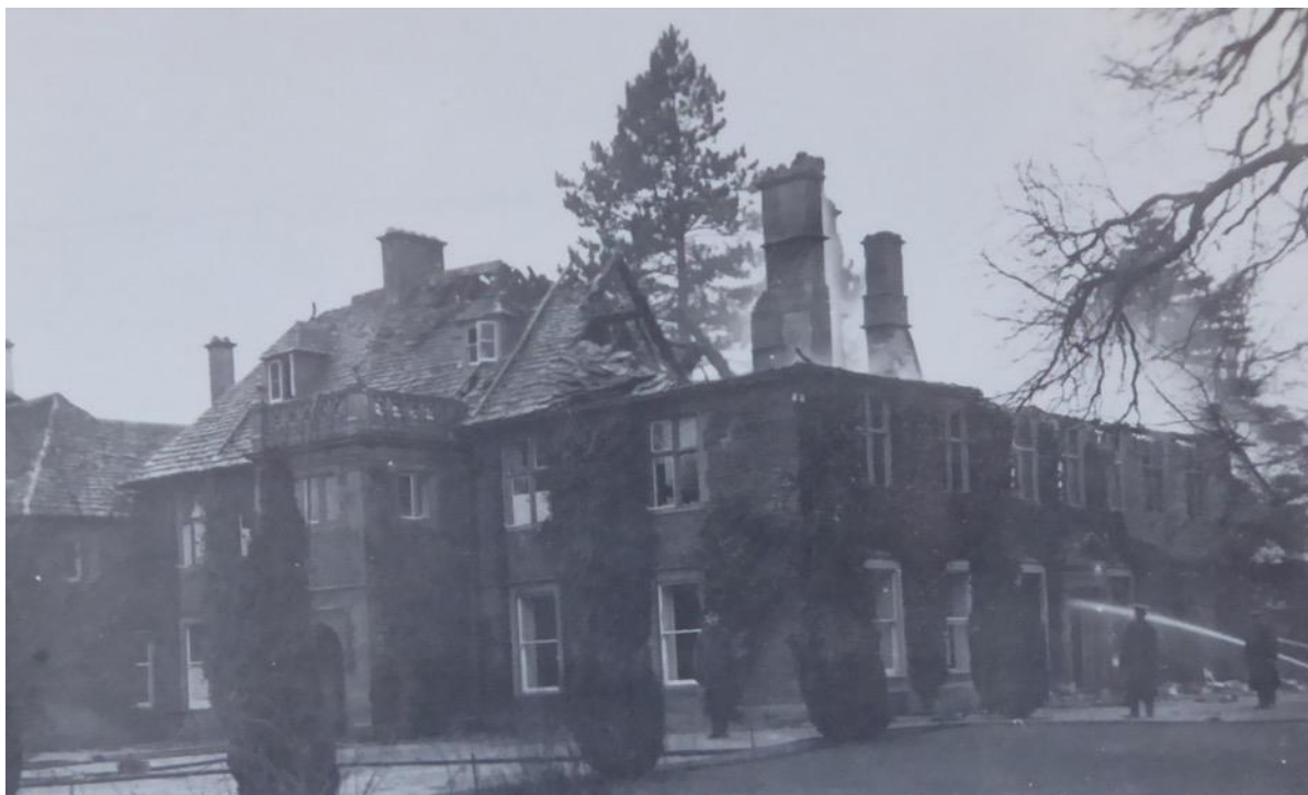
Figure C5: Melksham House 1920; immediate post-fire east elevation
