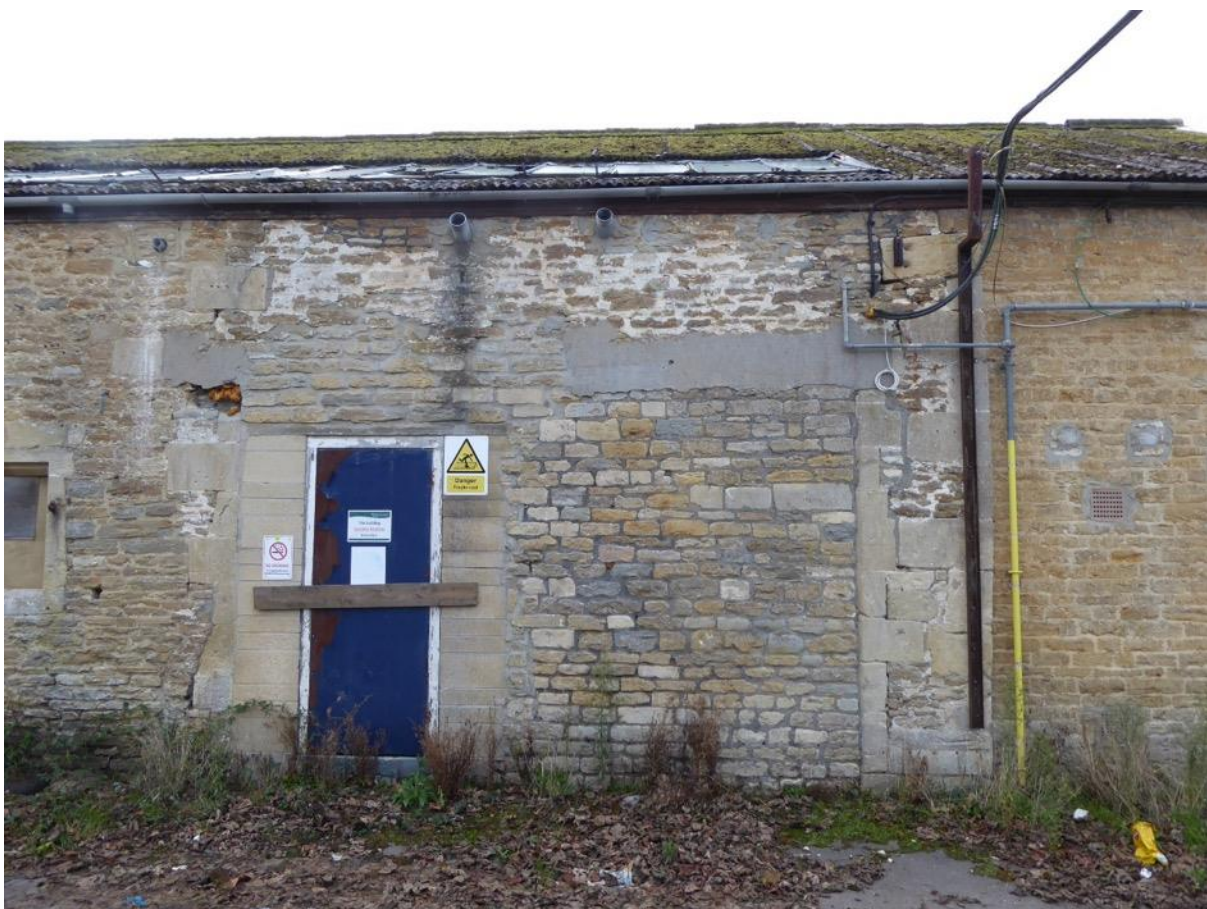
Figure 31: Former stable, former carriage opening now blocked
