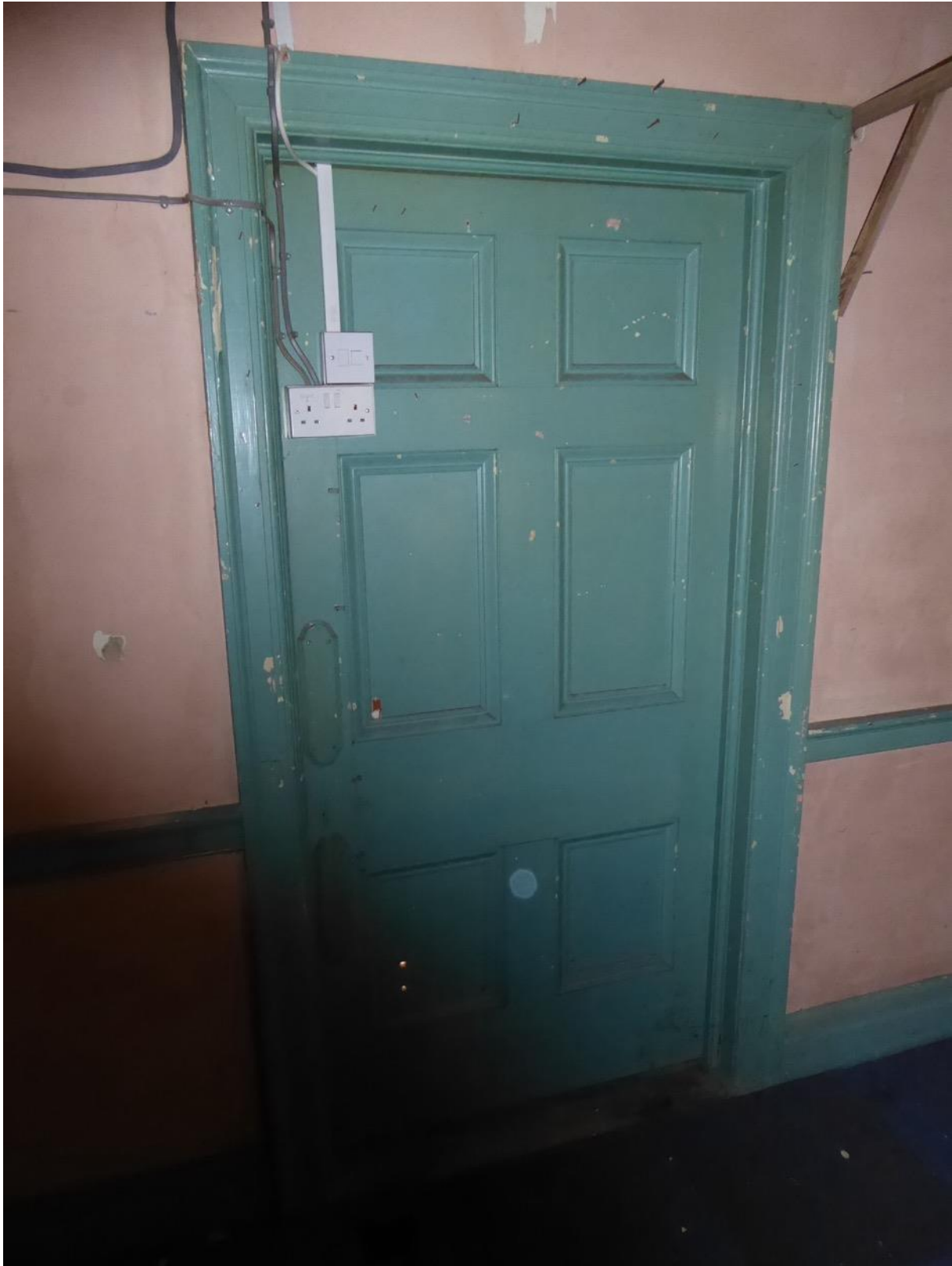
Figure 25: Six panel door – probably reproduction but possibly 18 th century with moulded architrave
