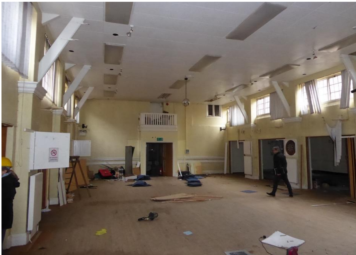
Figure 13: Concert hall (looking east)
