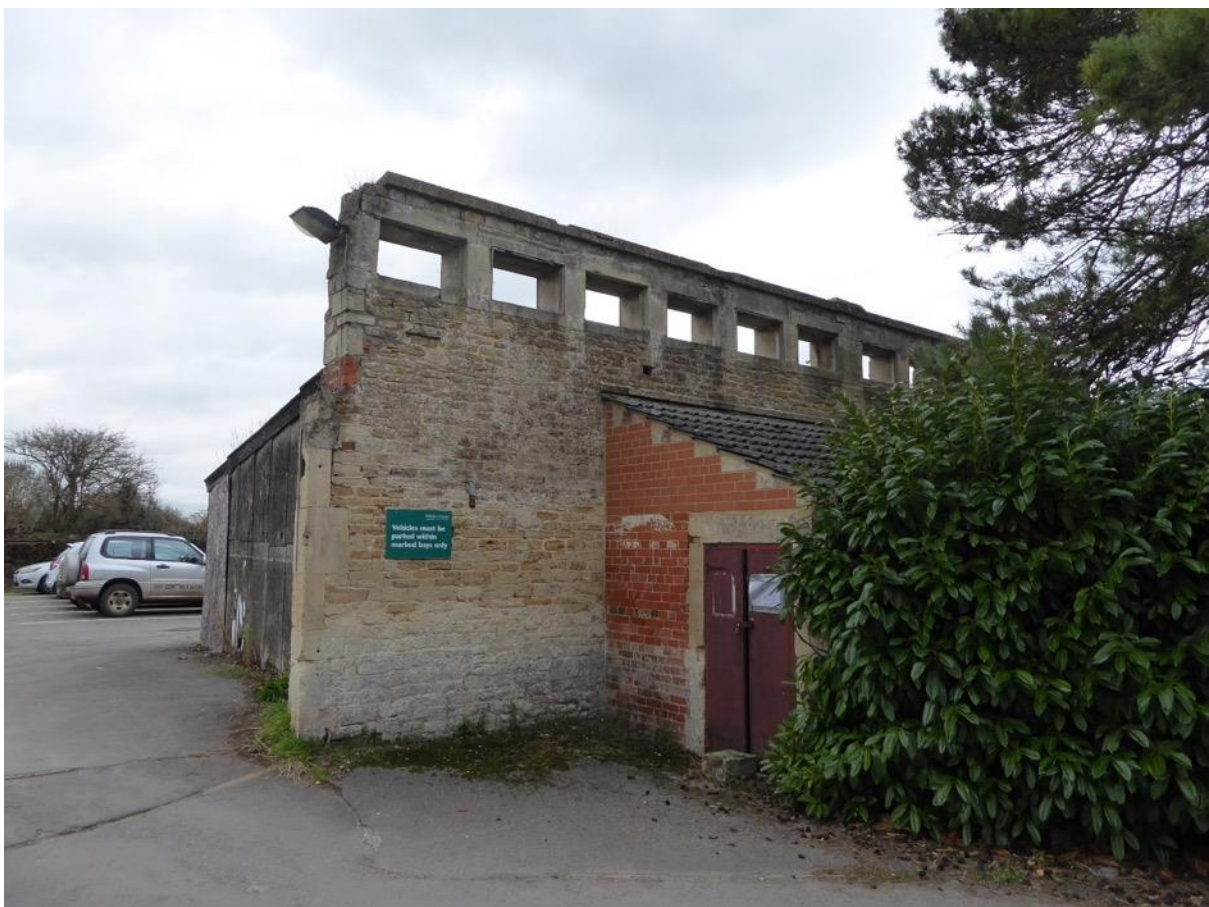
Figure 38: Possible former heated wall to former peach house to south-east of house
