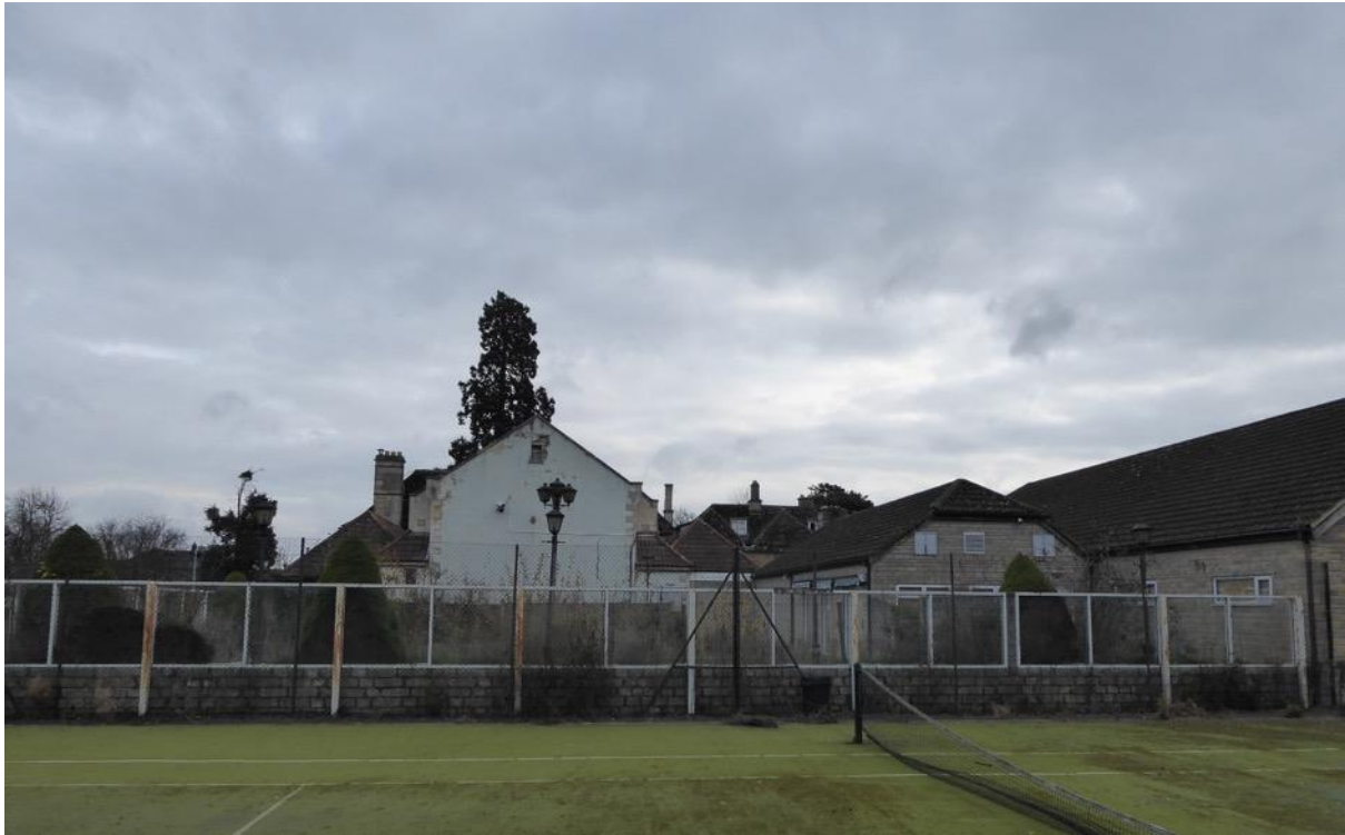
Figure 10: West elevation from tennis courts
