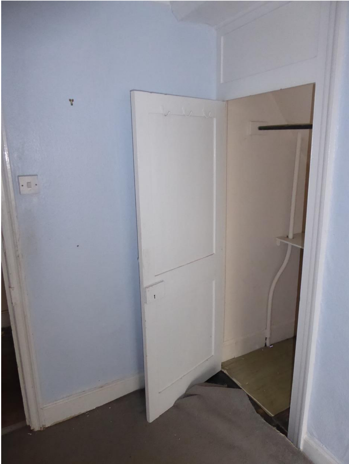
Figure 26: Simple two-panel late-18 th /early 19 th century door (probably re-used)
