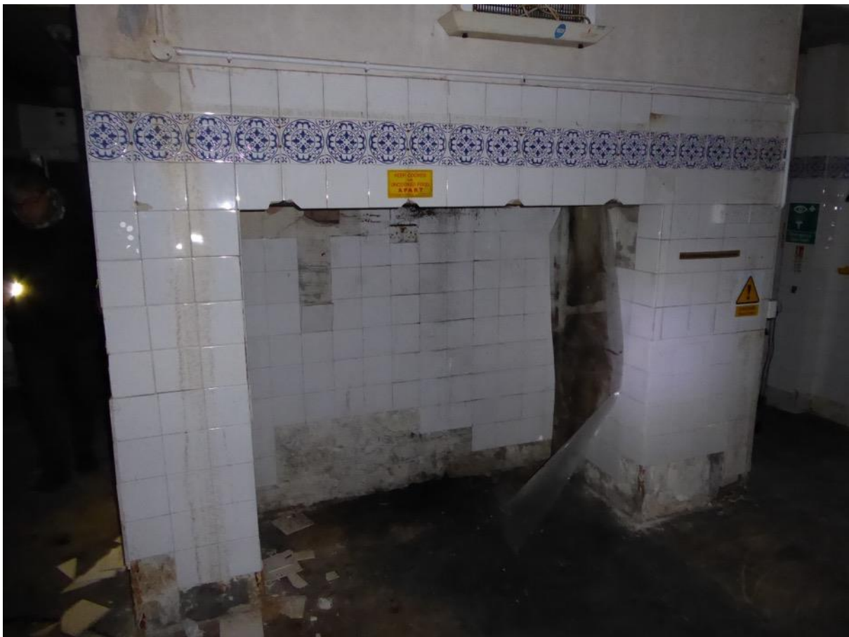
Figure 19: Kitchen fireplace (probably 17 th century in origin)
