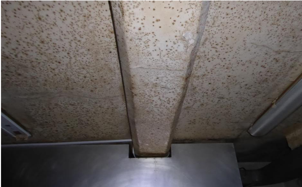
Figure 18: Chamfered beam to former kitchen
