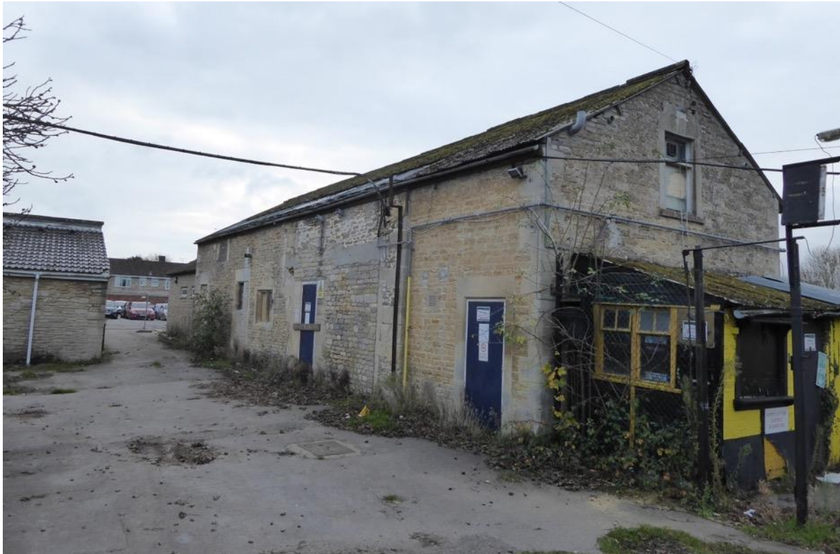
Figure 30: Former stable (now clubhouse) to south of house -north elevation
