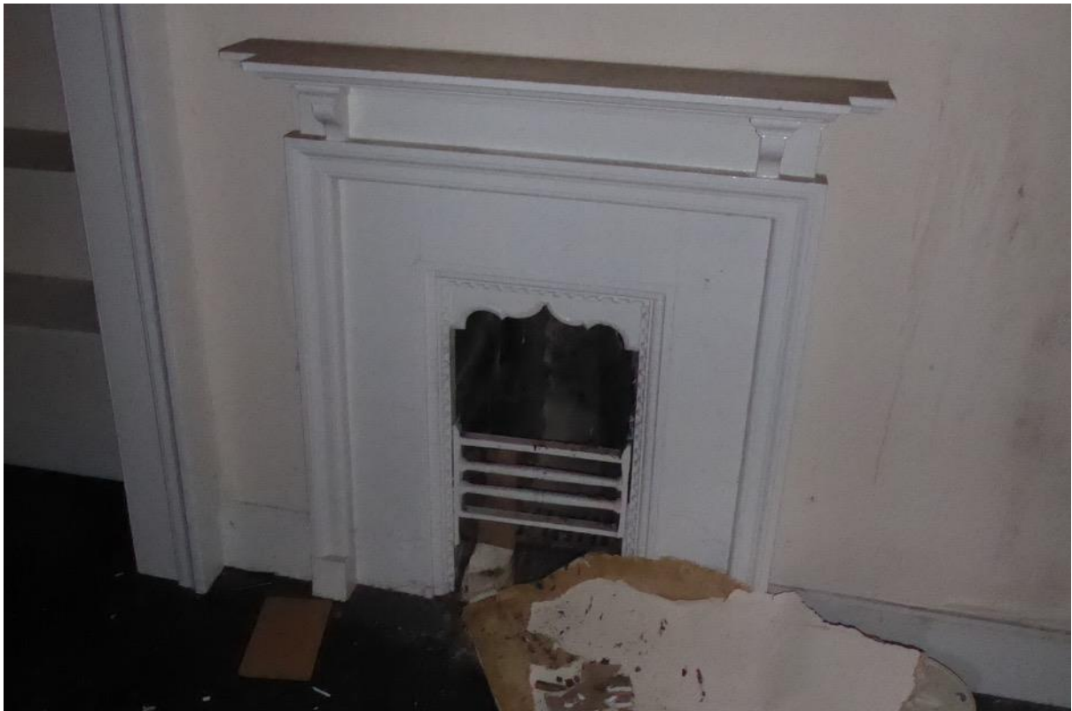
Figure 24: Late 19 th /early 20 th century fireplace, first floor central section of north-south range
