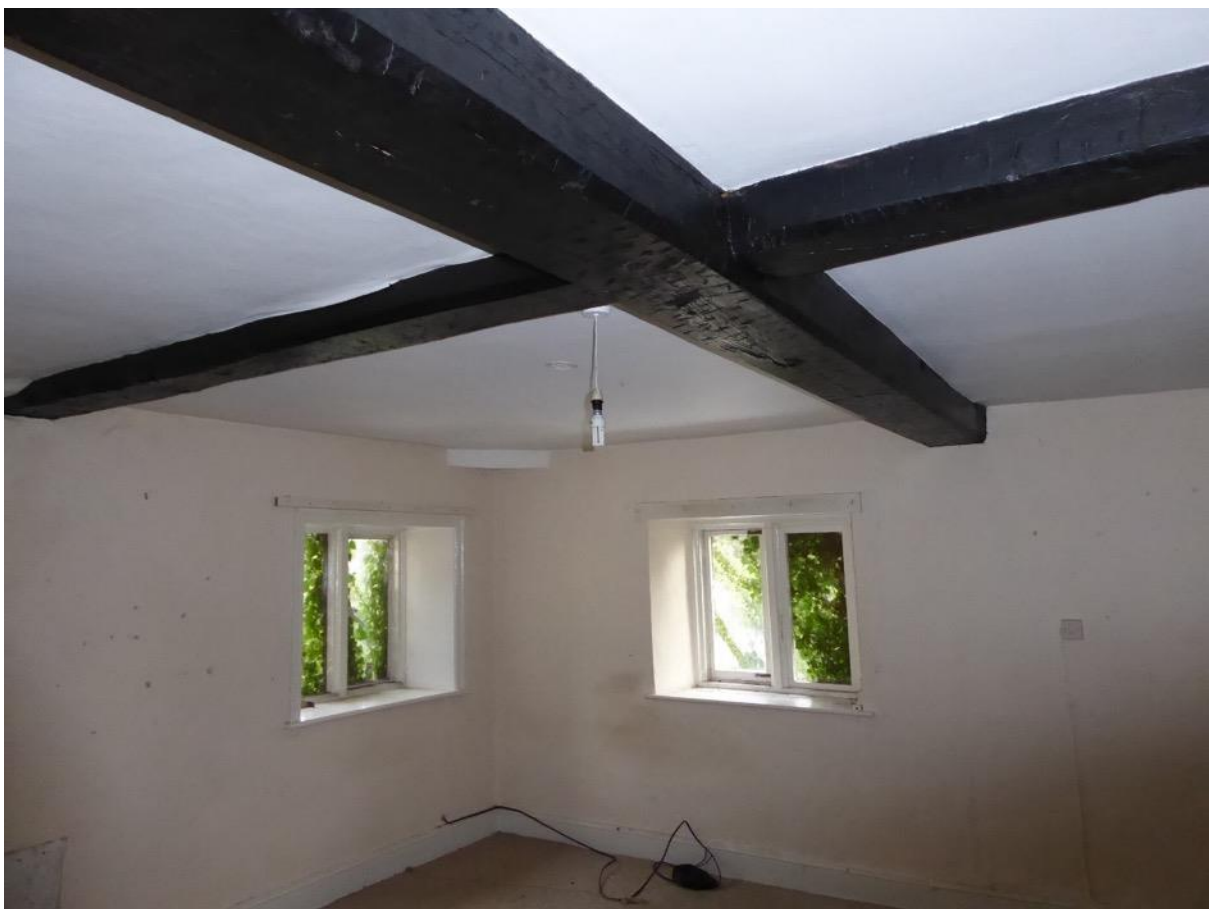
Figure 21: Ceiling beams to room above kitchen
