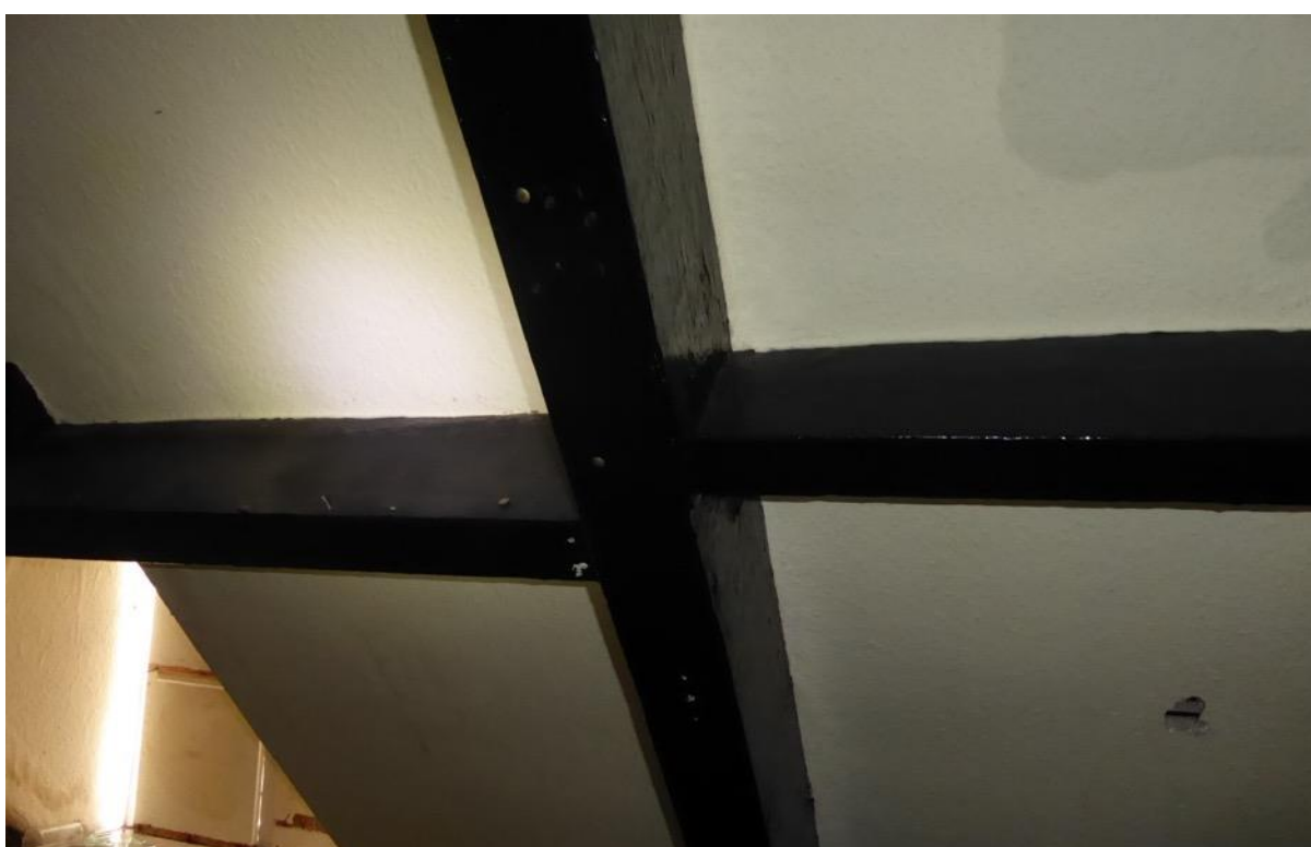
Figure 29: Staggered purlin to attic above Central section of north-south range (north section)
