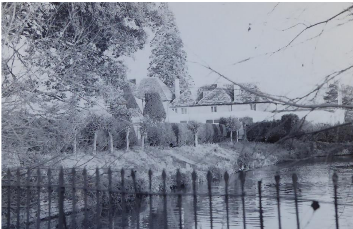
Figure C12: West elevation from the ornamental lake looking north-east c1977
