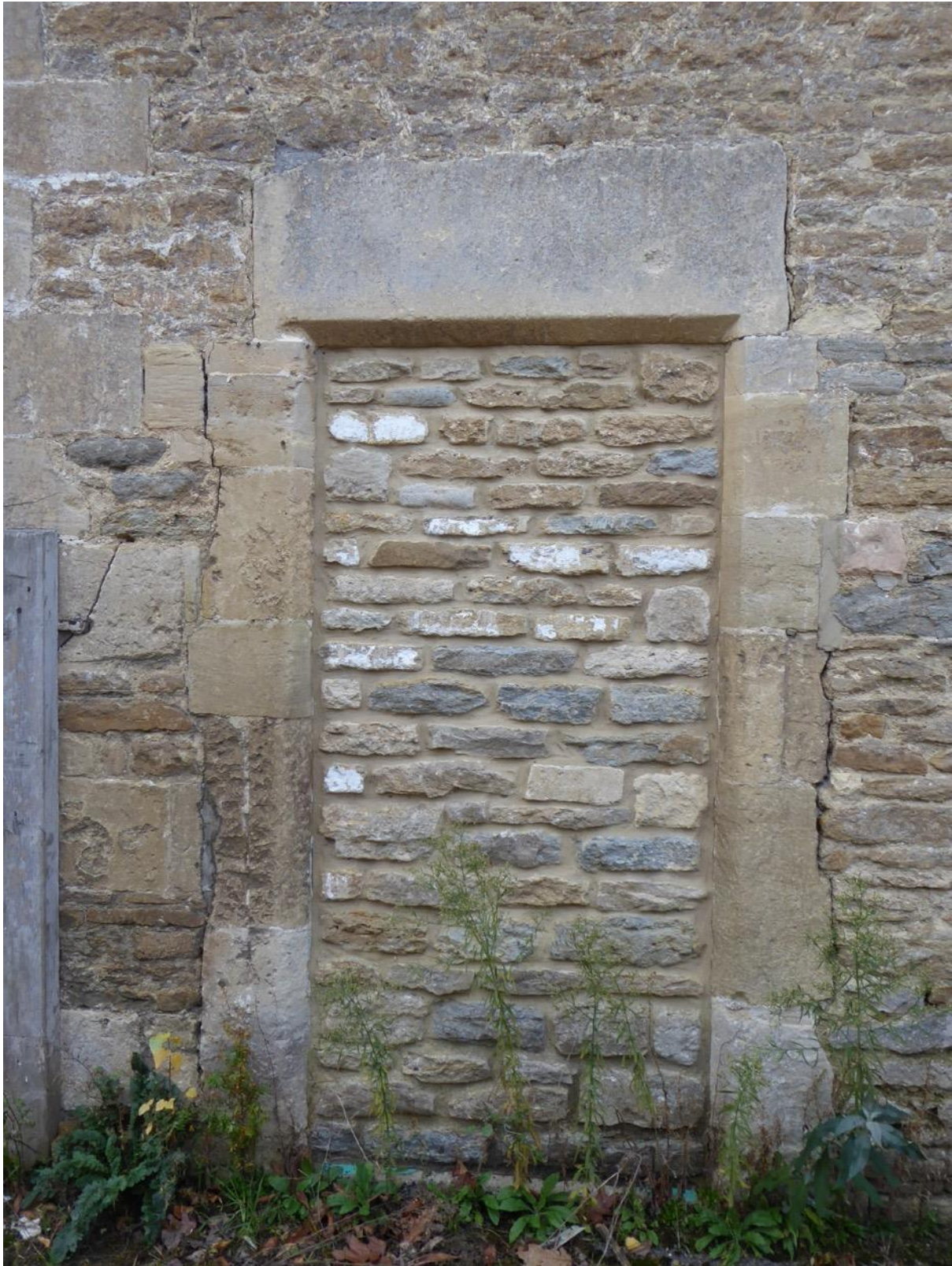
Figure 32: Possible re-used 17 th century chamfered door opening, now blocked
