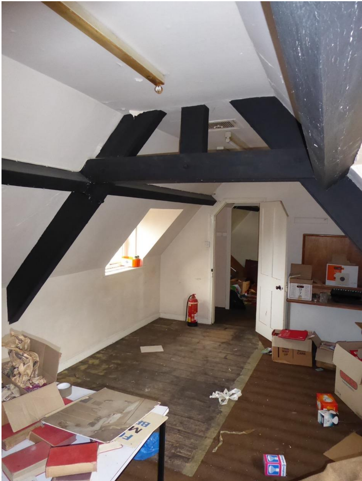
Figure 27: Exposed roof to attic – in line purlins (to central section)
