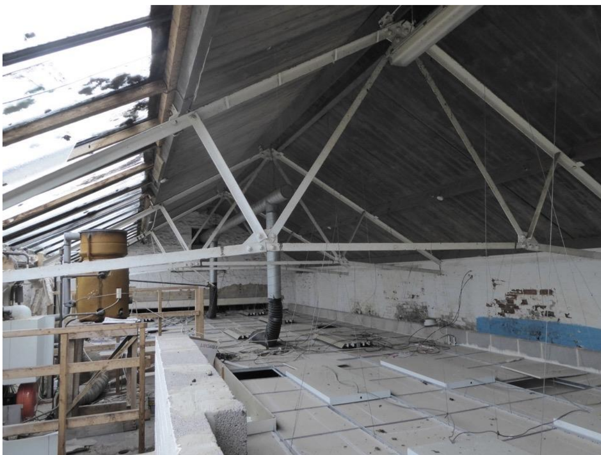
Figure 36: Former stable – first floor and roof
