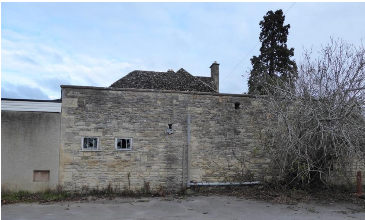
Figure 11: South elevation (former service yard)
