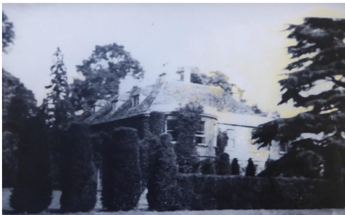
Figure C2: Melksham House c1900 (north and west elevations)
