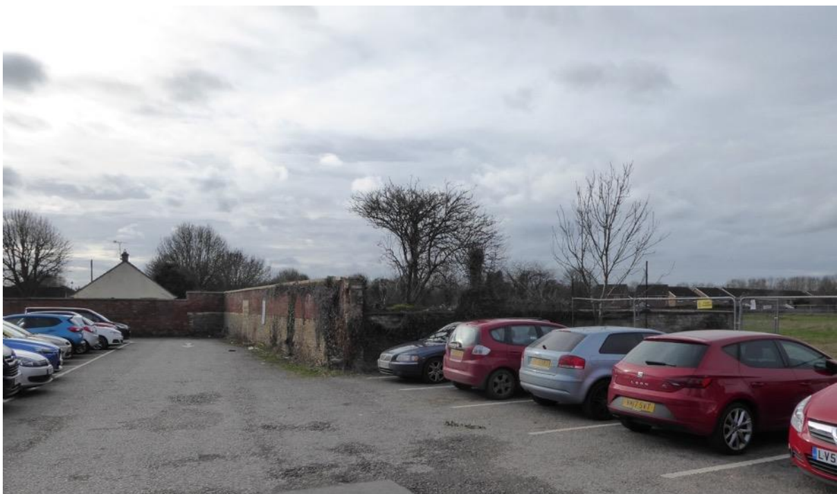
Figure 40: Remnant section of former kitchen garden walls (now enclosing car park)
