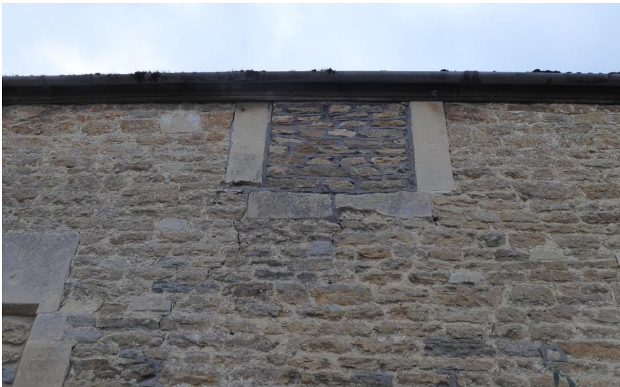
Figure 34: Blocked stone opening
